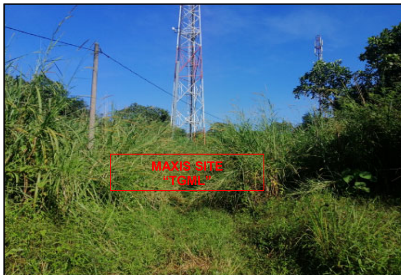
LOCATION AT SITE TGML
