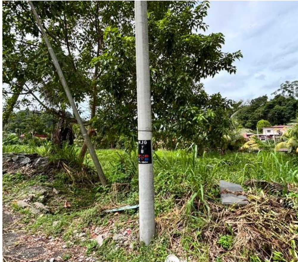
GAMBAR 6: TIANG TNB DI CH5100 (5.42562°N, 101.12465°E)
