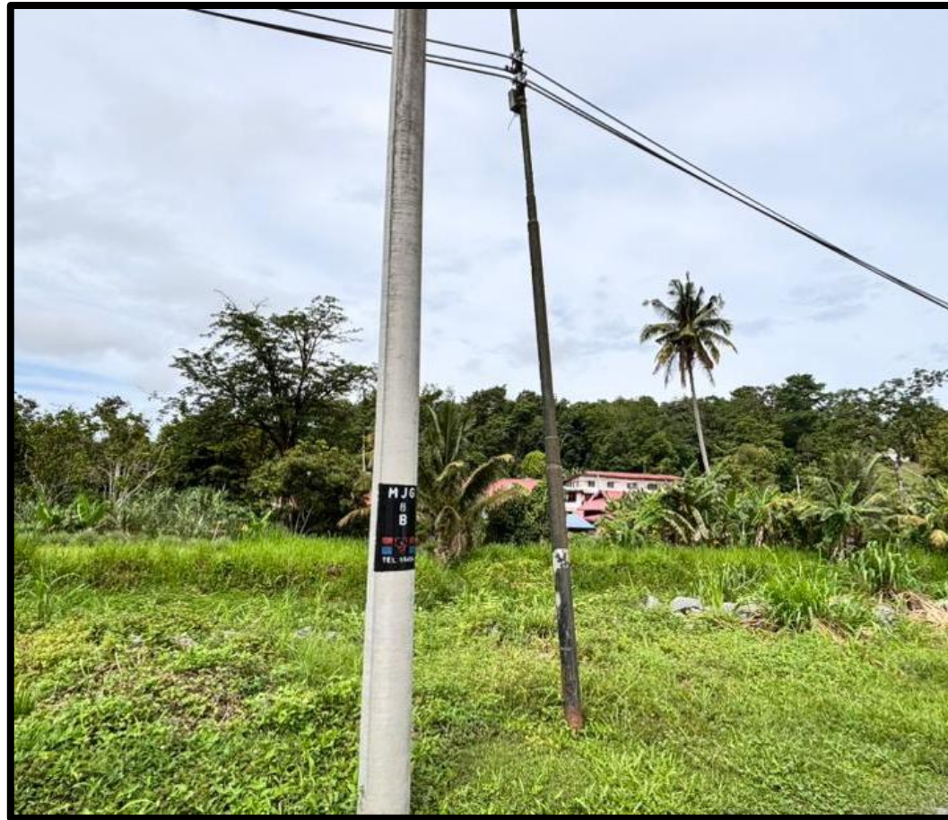
GAMBAR 7: TIANG TNB DI CH5000 (5.42550°N, 101.12496°E)
