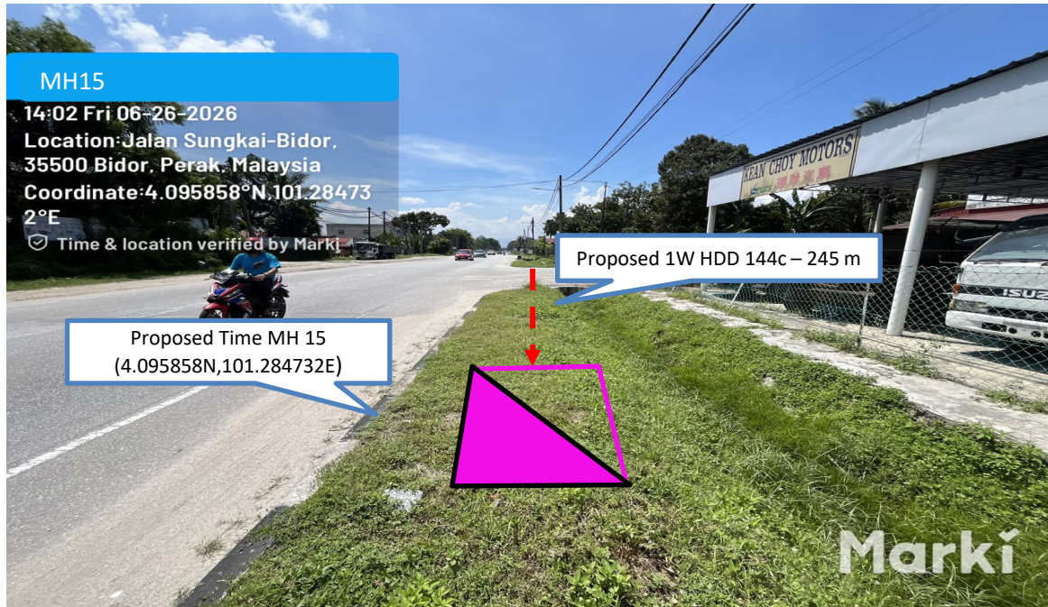
Prop 1W HDD 144C from Proposed Time MH14 to Proposed Time MH15 – 245 m
