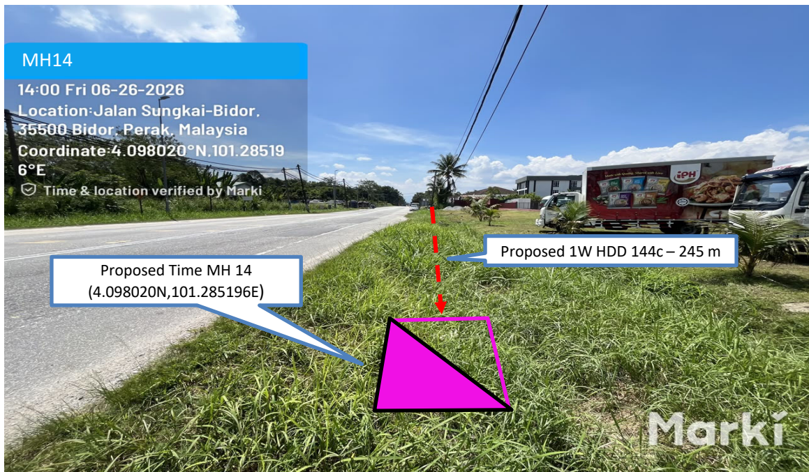
Prop 1W HDD 144C from Proposed Time MH13 to Proposed Time MH14 – 245 m
