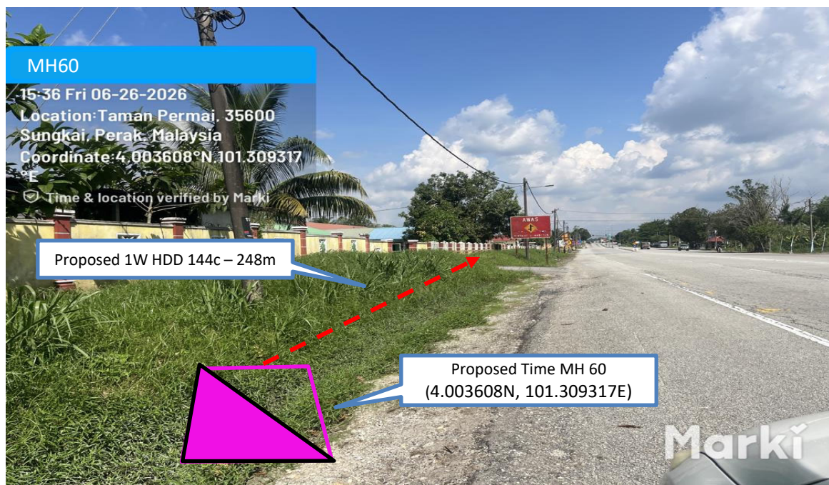
Prop 1W HDD 144C from Proposed Time MH60 n to Proposed Time MH61–248 m
