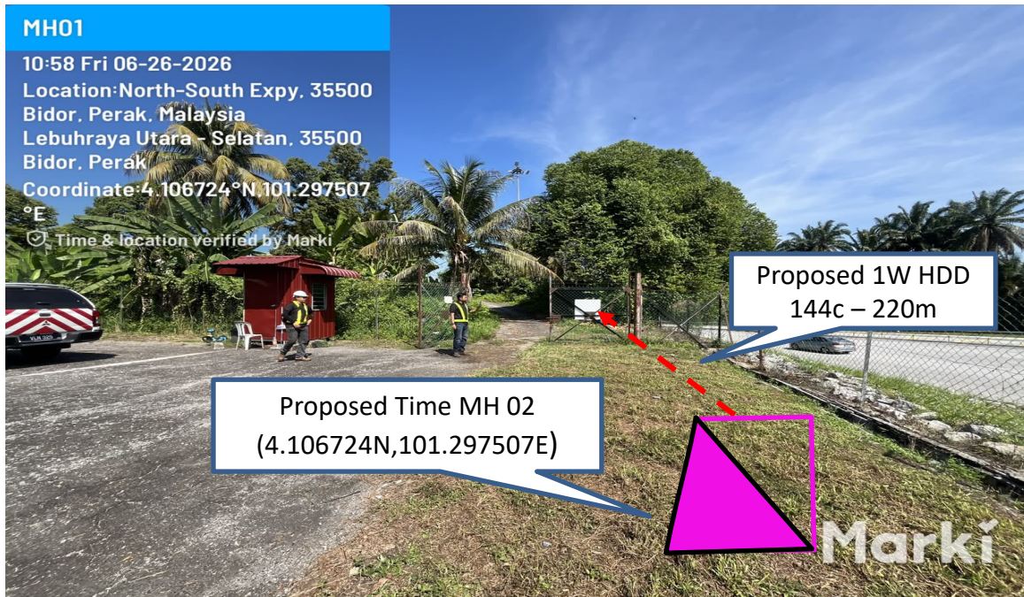
Prop 1W HDD 144C from Proposed Time MH01 to Proposed Time MH02 – 220 m
