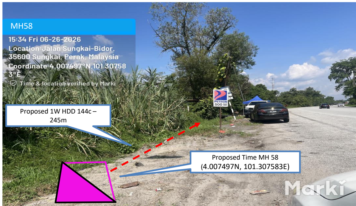
Prop 1W HDD 144C from Proposed Time MH58 to Proposed Time MH59– 245 m
