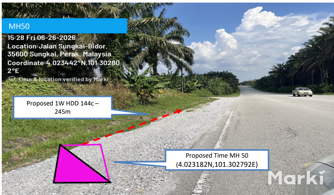
Prop 1W HDD 144C from Proposed Time MH49 to Proposed Time MH50– 245 m
