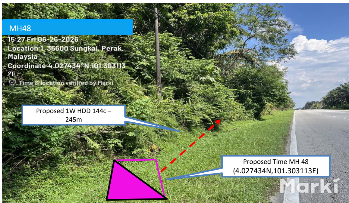
Prop 1W HDD 144C from Proposed Time MH48 to Proposed Time MH49– 245 m
