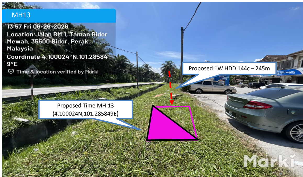
Prop 1W HDD 144C from Proposed Time MH12 to Proposed Time MH13 – 245 m
