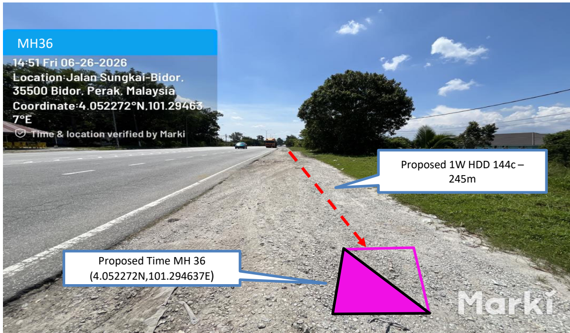
Prop 1W HDD 144C from Proposed Time MH35 to Proposed Time MH36– 245 m
