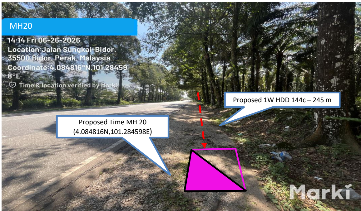
Prop 1W HDD 144C from Proposed Time MH19 to Proposed Time MH20 – 245 m
