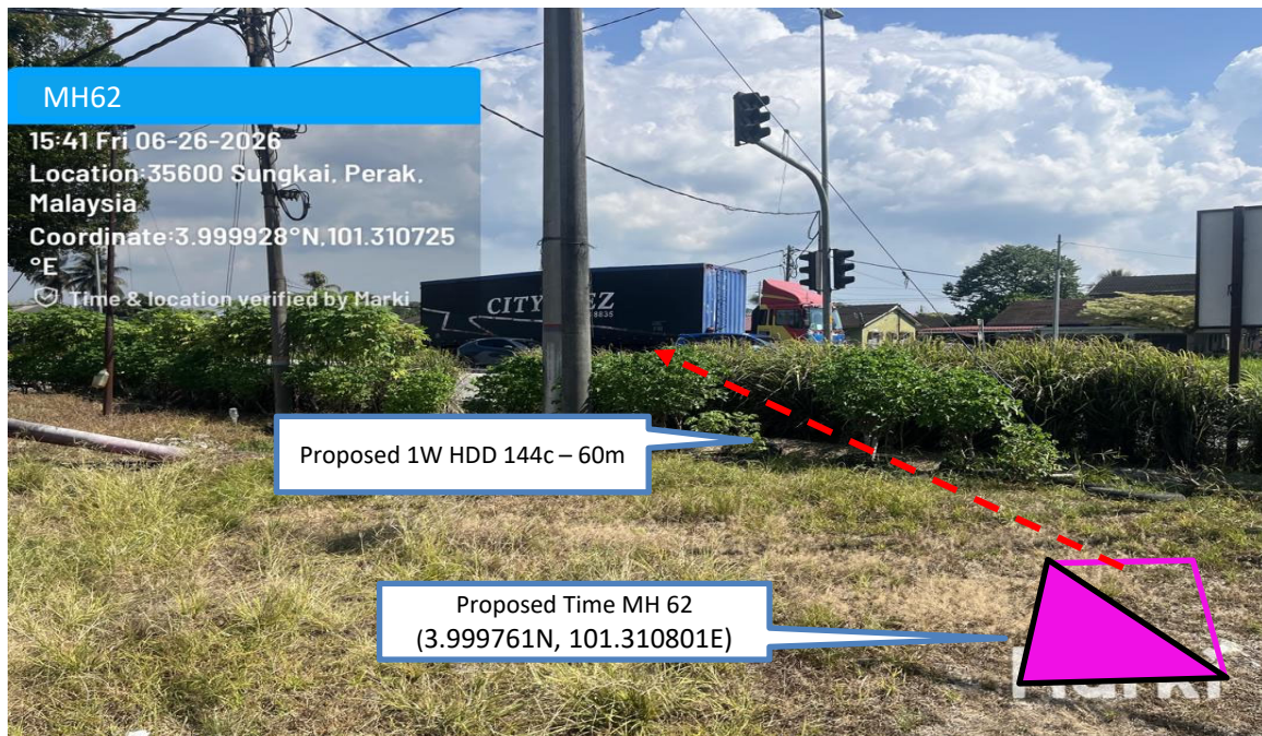
Prop 1W HDD 144C from Proposed Time MH62 n to Proposed Existing Time Manhole– 60 m
