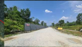
SIDE CONDITION - CONSTRUCTION ROAD/ACCESS
