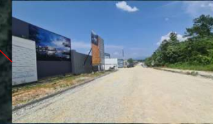
SIDE CONDITION - CONSTRUCTION ROAD/ACCESS
