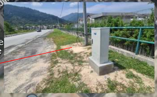
EXISTING TM OVERHEAD LINE
