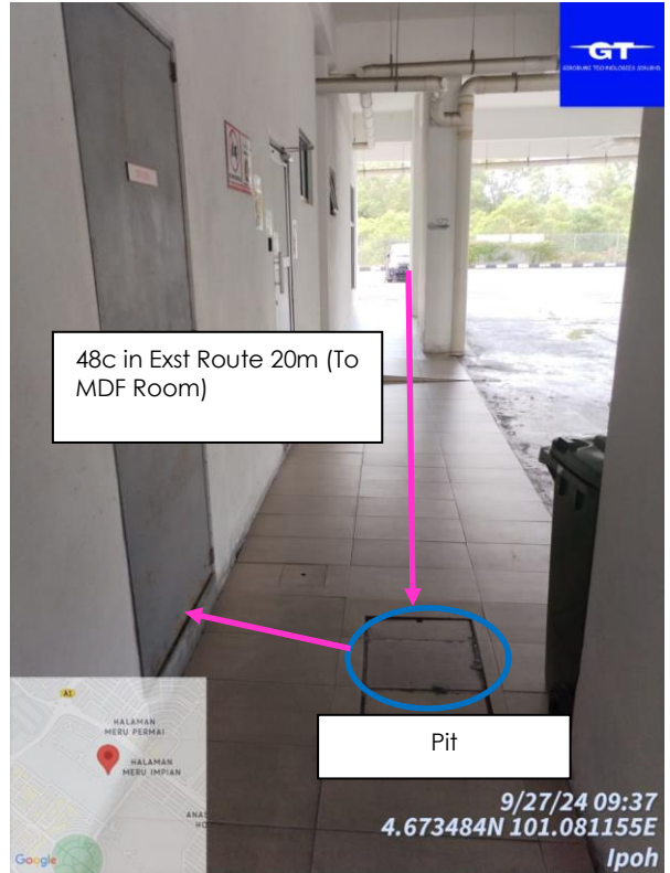
Propose route at Jalan Meru Impian - Fiber Pulling method
