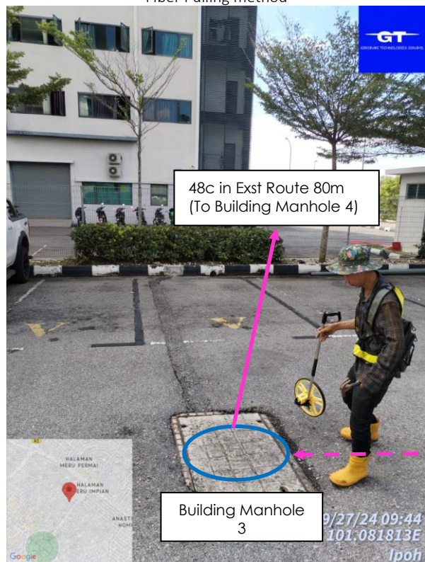
Propose route at Jalan Meru Impian - Fiber Pulling method
