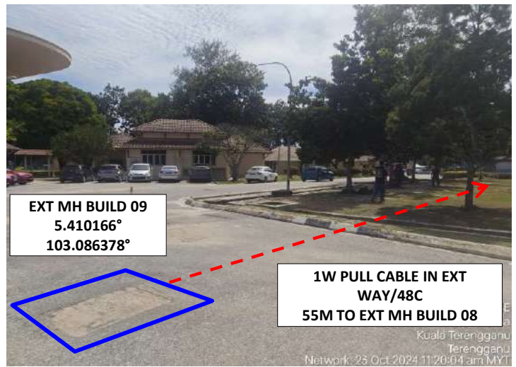
Propose route in UMT's Compound – Pull Cable method
