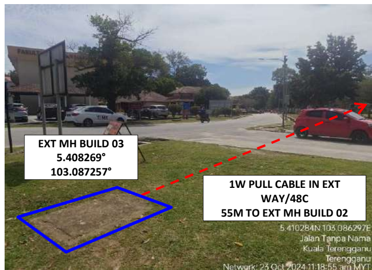
Propose route in UMT's Compound – Pull Cable method
