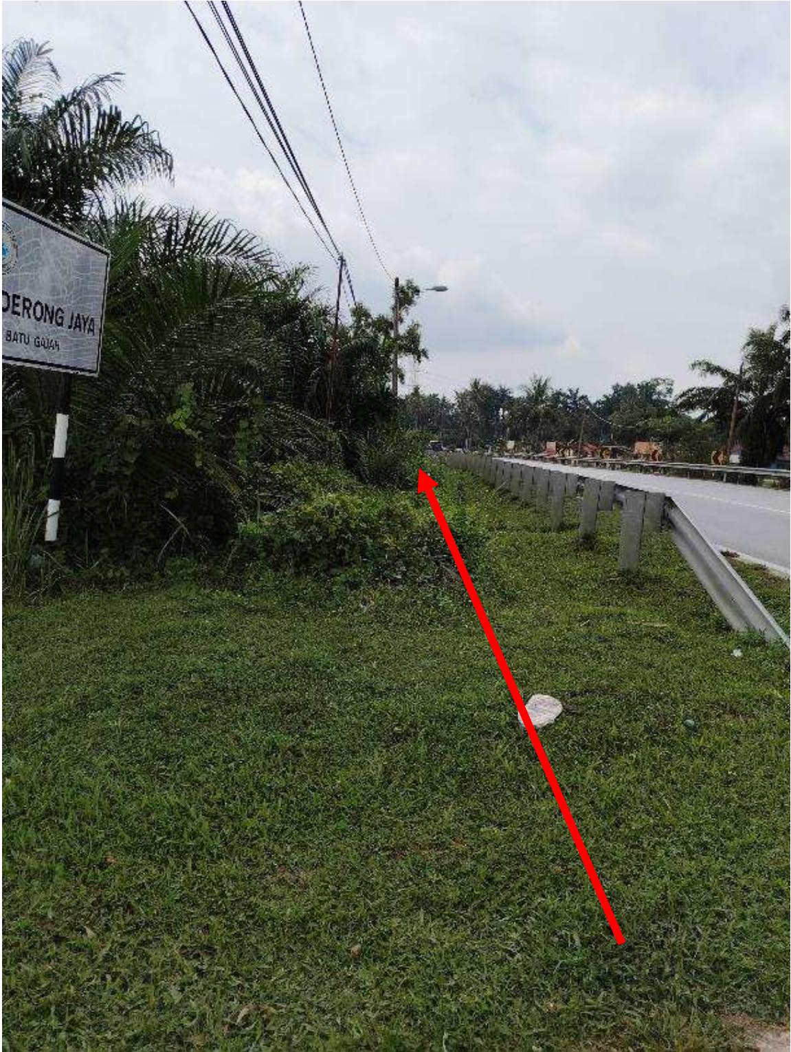
JALAN TG TUALANG (A15) -HDD
