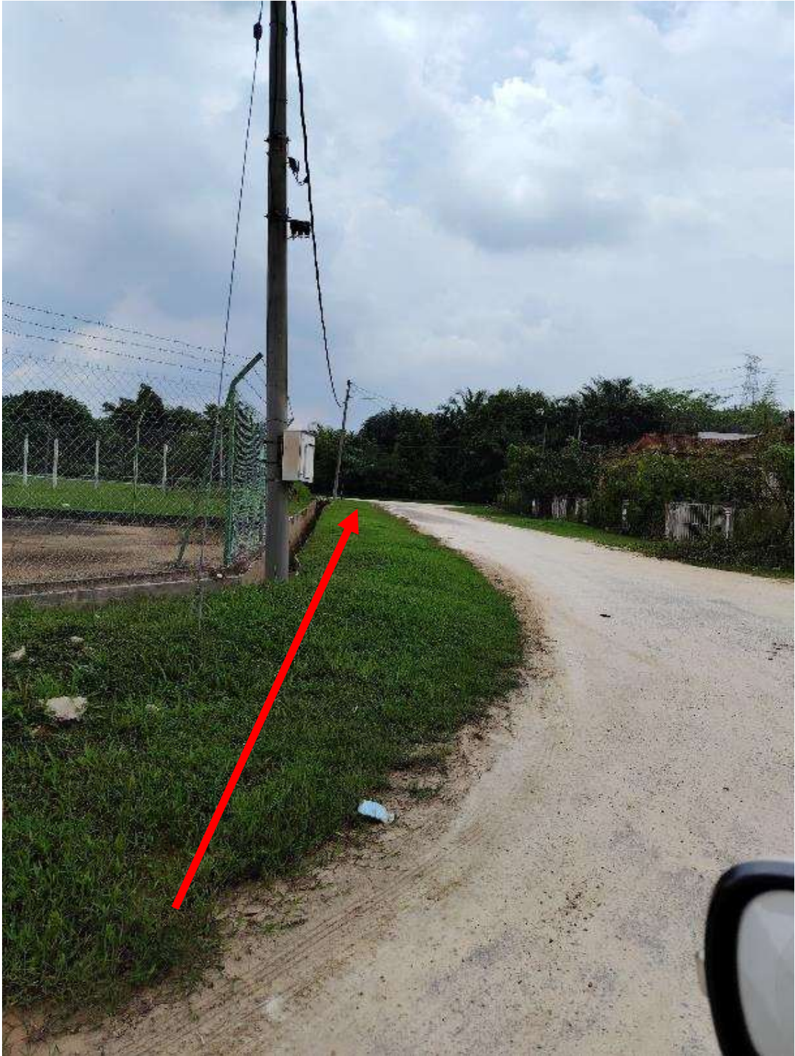
JALAN CHENDERONG 1-OPEN CUT
