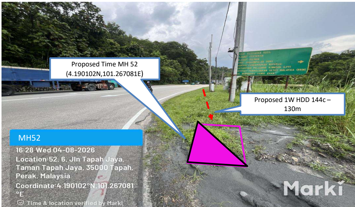
Prop 1W HDD 144C from Proposed Time MH51 n to Proposed Time MH52- 130 m
