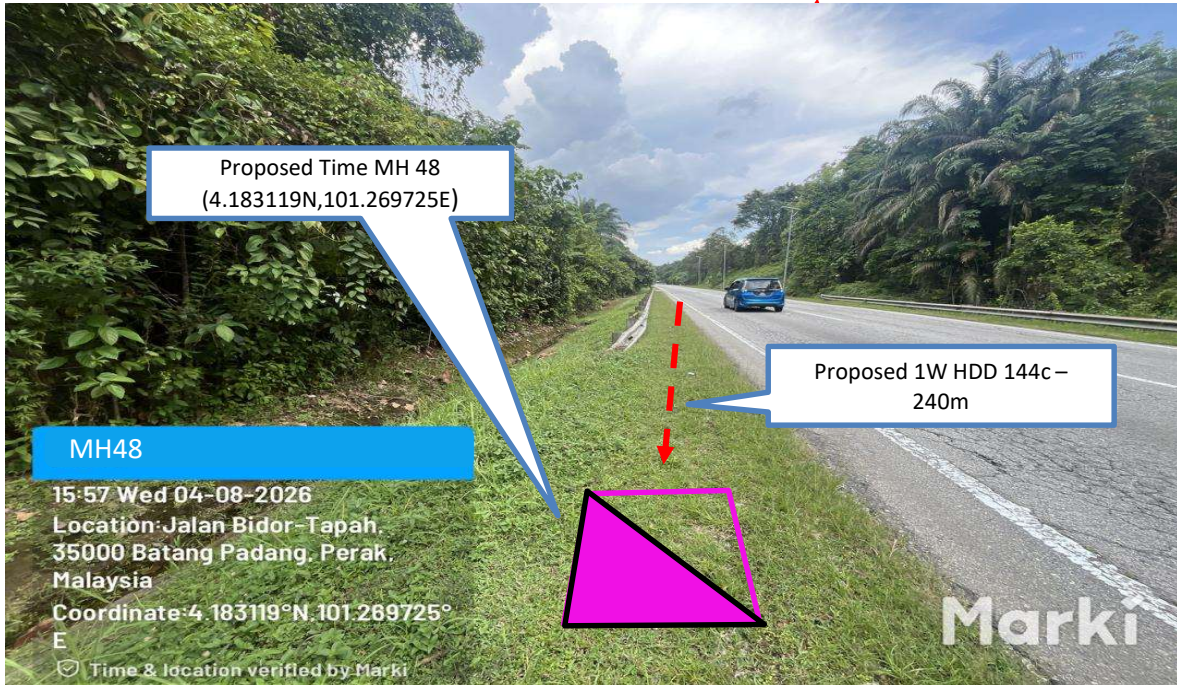
Prop 1W HDD 144C from Proposed Time MH47 n to Proposed Time MH48– 240 m
