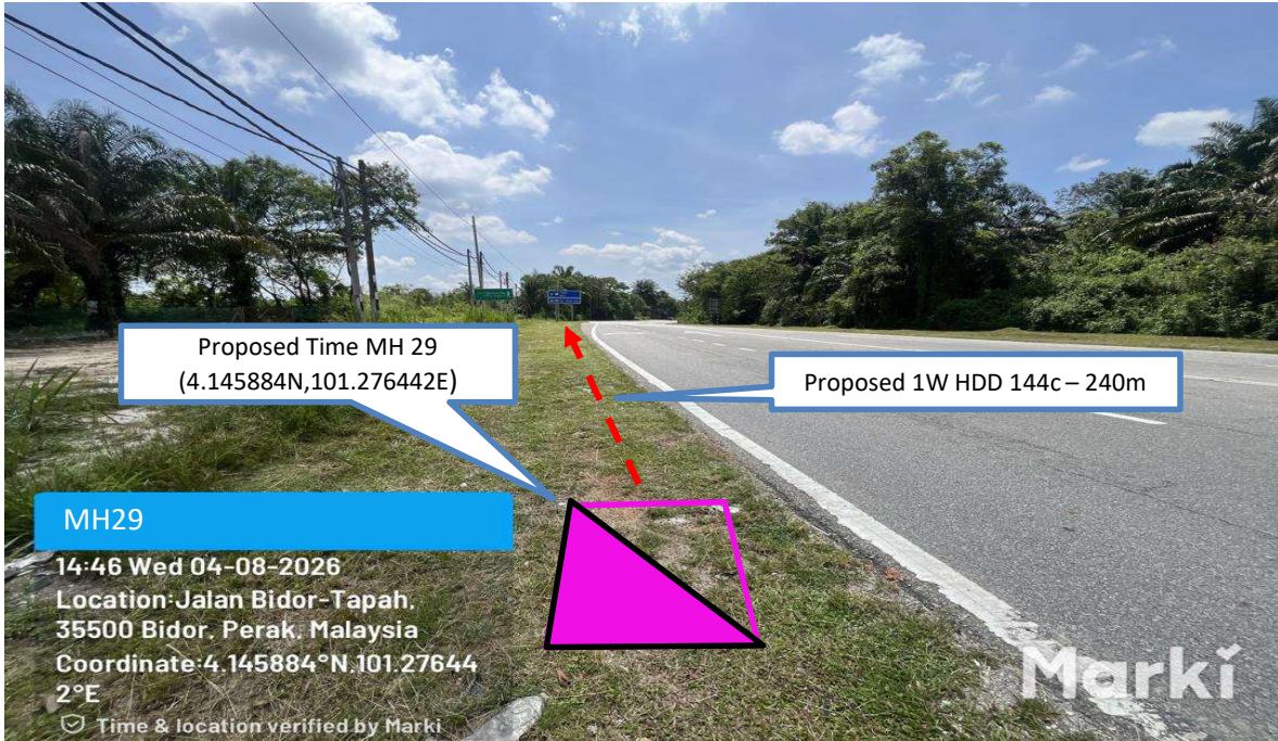
Prop 1W HDD 144C from Proposed Time MH28 n to Proposed Time MH29 – 240 m
