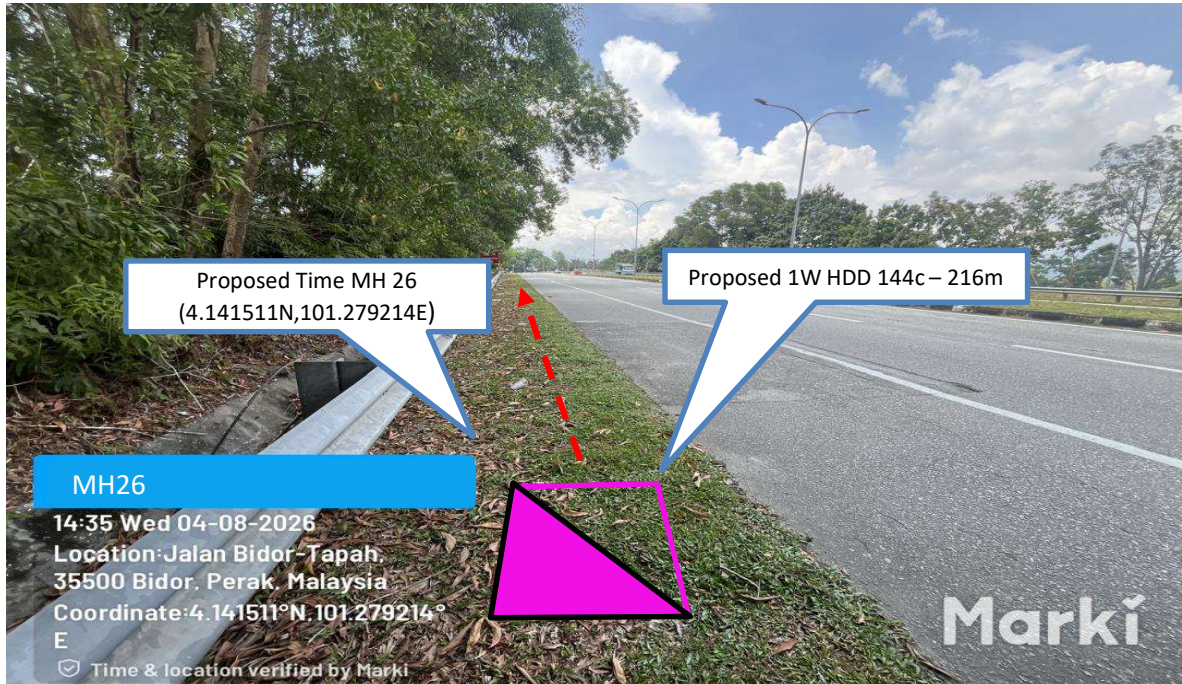
Prop 1W HDD 144C from Proposed Time MH25 n to Proposed Time MH26 – 216 m
