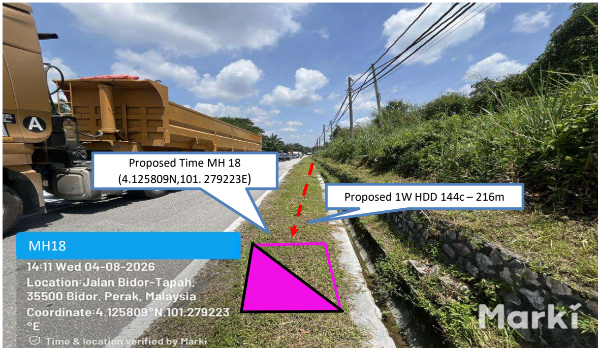
Prop 1W HDD 144C from Proposed Time MH17 n to Proposed Time MH18 – 216 m
