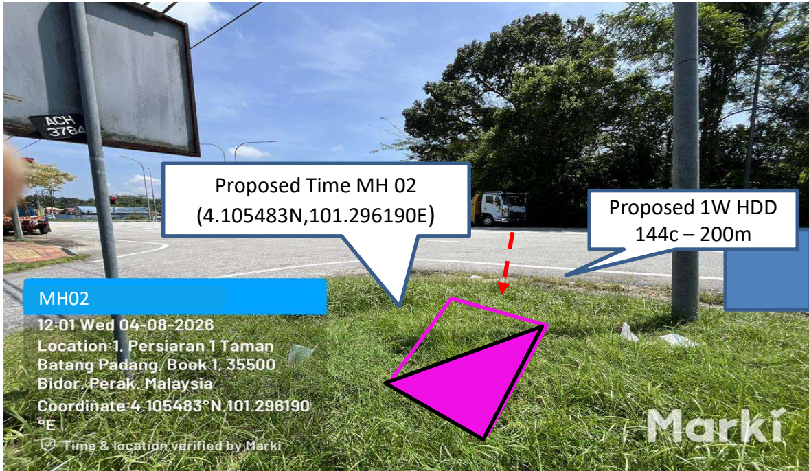
Prop 1W HDD 144C from Proposed Time MH01 to Proposed Time MH02 – 200 m
