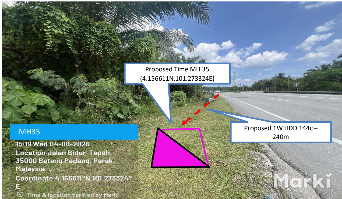
Prop 1W HDD 144C from Proposed Time MH34 n to Proposed Time MH35- 240 m
