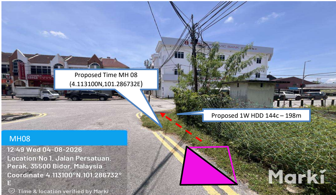
Prop 1W HDD 144C from Proposed Time MH07 n to Proposed Time MH08 - 198 m
