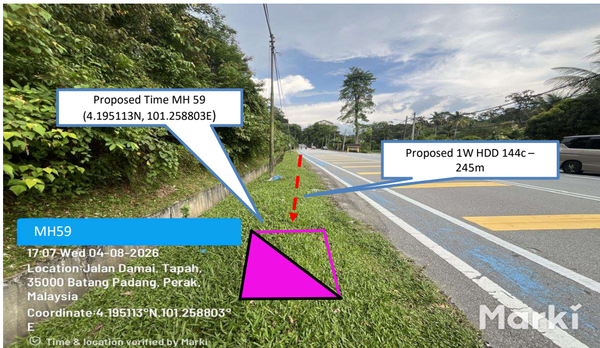
Prop 1W HDD 144C from Proposed Time MH58 n to Proposed Time MH59–245m
