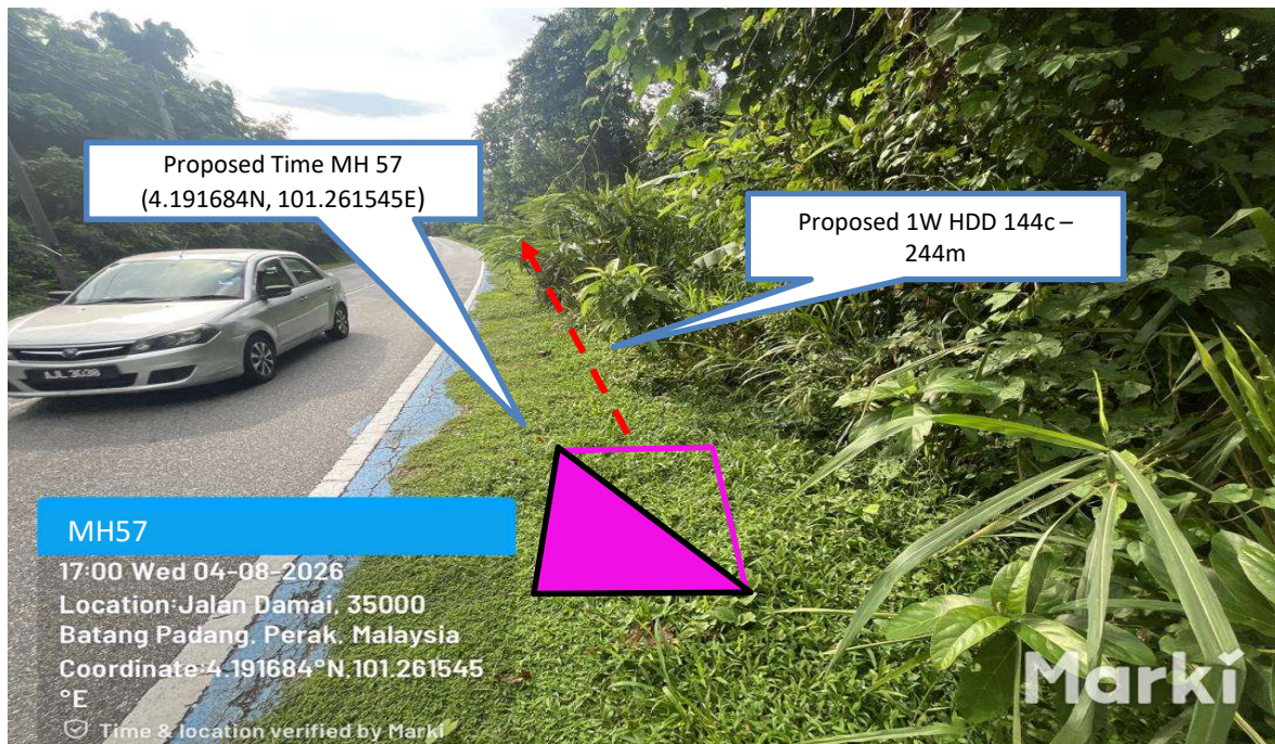
Prop 1W HDD 144C from Proposed Time MH57 n to Proposed Time MH58-244m
