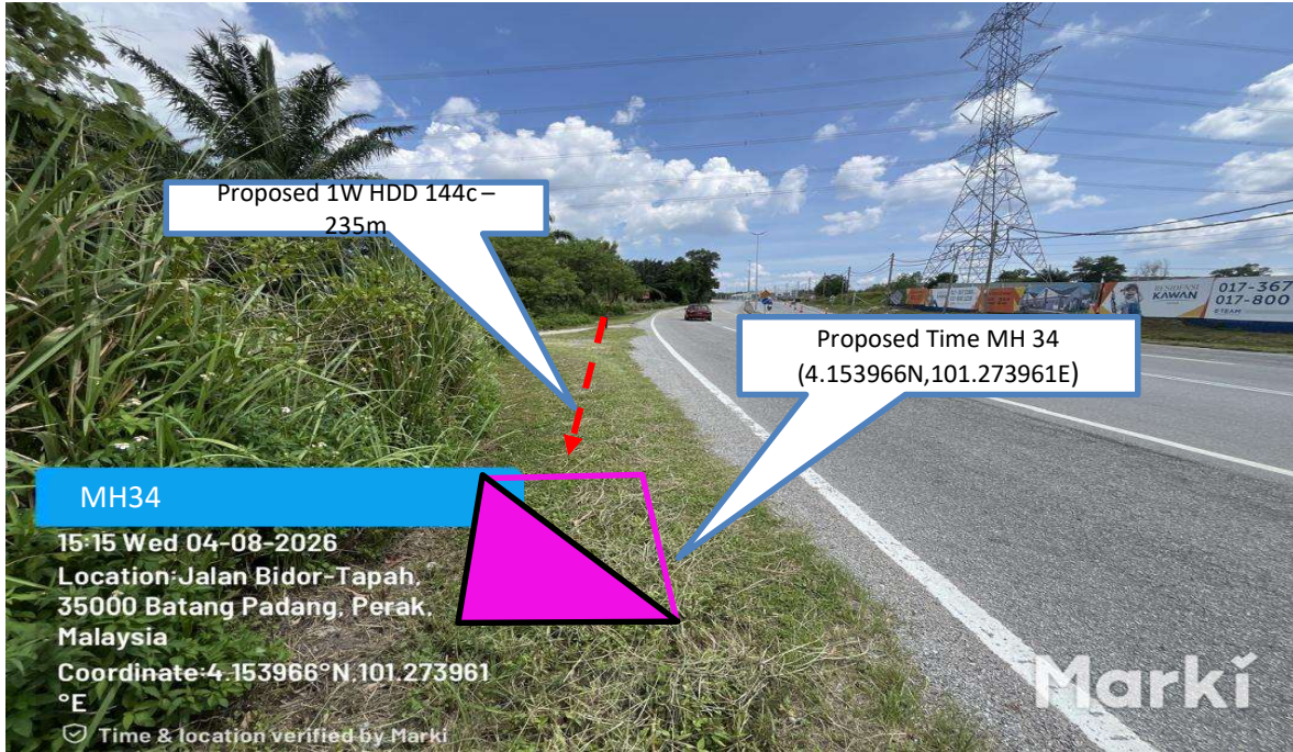
Prop 1W HDD 144C from Proposed Time MH33 n to Proposed Time MH34 - 235 m
