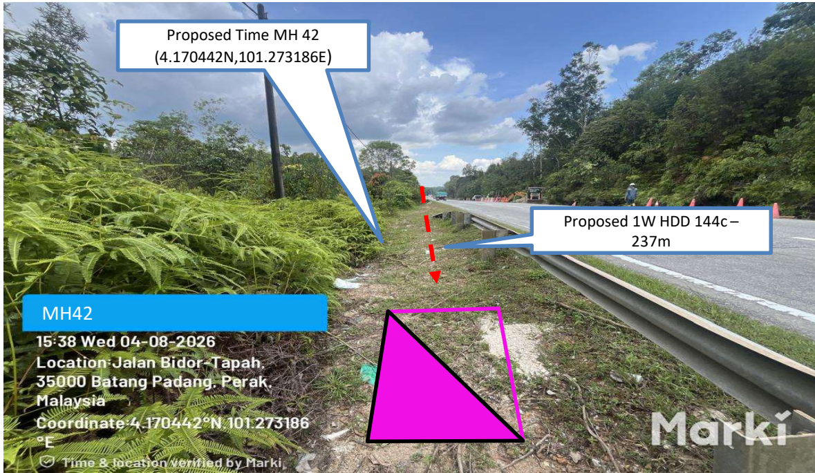
Prop 1W HDD 144C from Proposed Time MH41 n to Proposed Time MH42– 237 m
