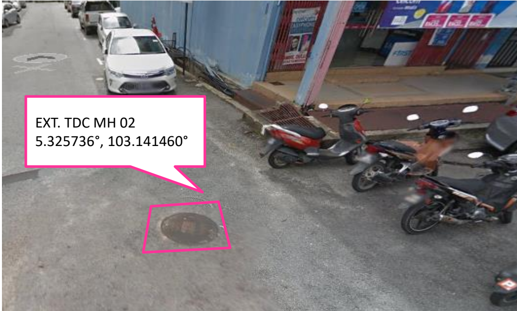
Existing TDC Manhole (MH 02 )
