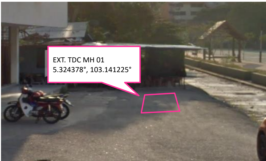
Existing TDC Manhole (MH 01 )
