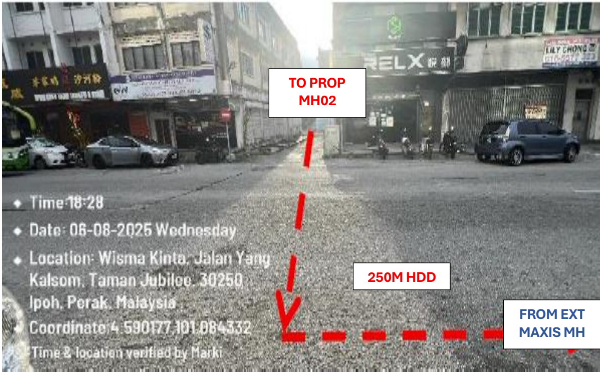
PICTURE 3 : PROPOSE 250M HDD TO PROP MH02
