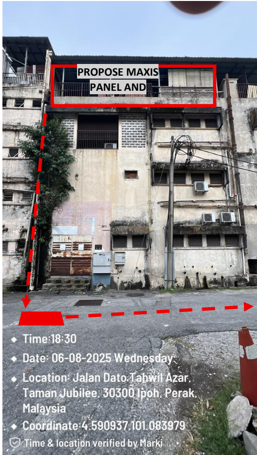
PICTURE 1 : UM T5 CABINET/ROOT TOP BUILDING PROPOSE GI PIPE, NEW MH AND 2 WAY HDD
