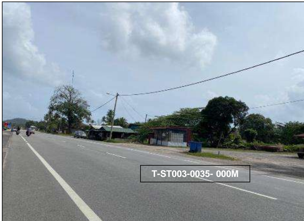
LOCATION AT JALAN KUALA TERENGGANU
