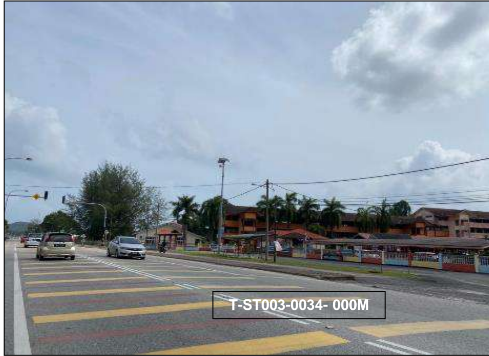
LOCATION AT JALAN KUALA TERENGGANU
