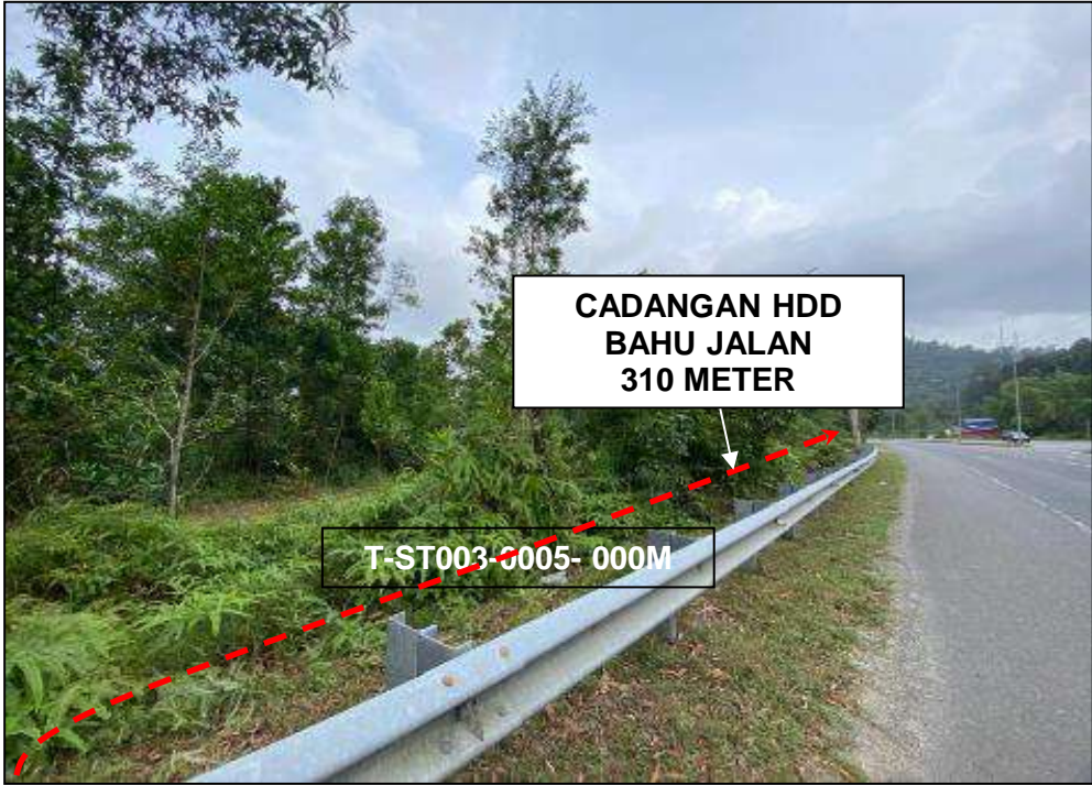
LOCATION AT JALAN PAKA
