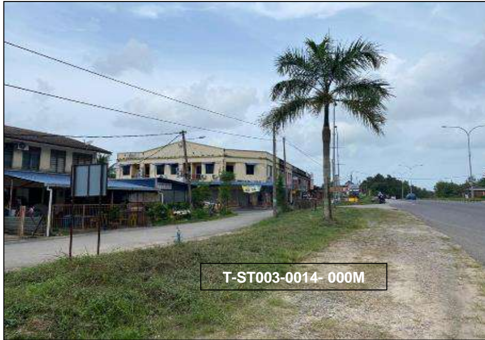
LOCATION AT JALAN PAKA
