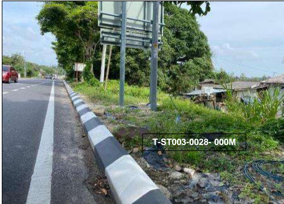
LOCATION AT JALAN KUALA TERENGGANU
