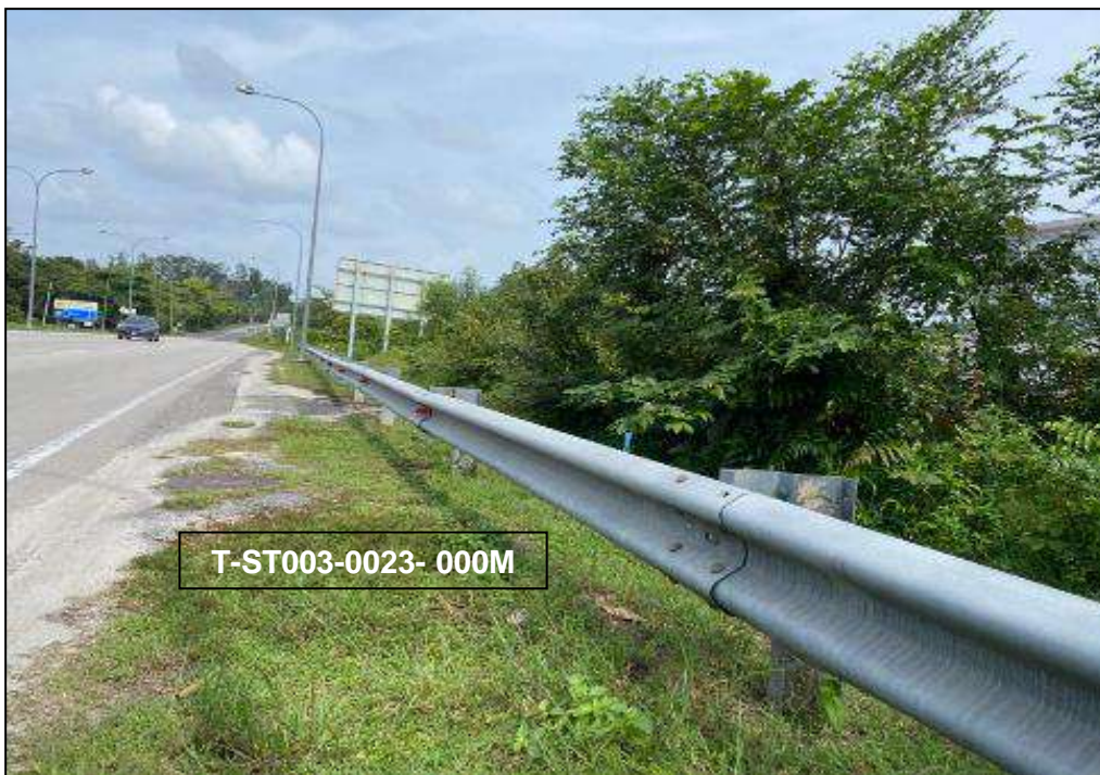
LOCATION AT JALAN KUALA TERENGGANU
