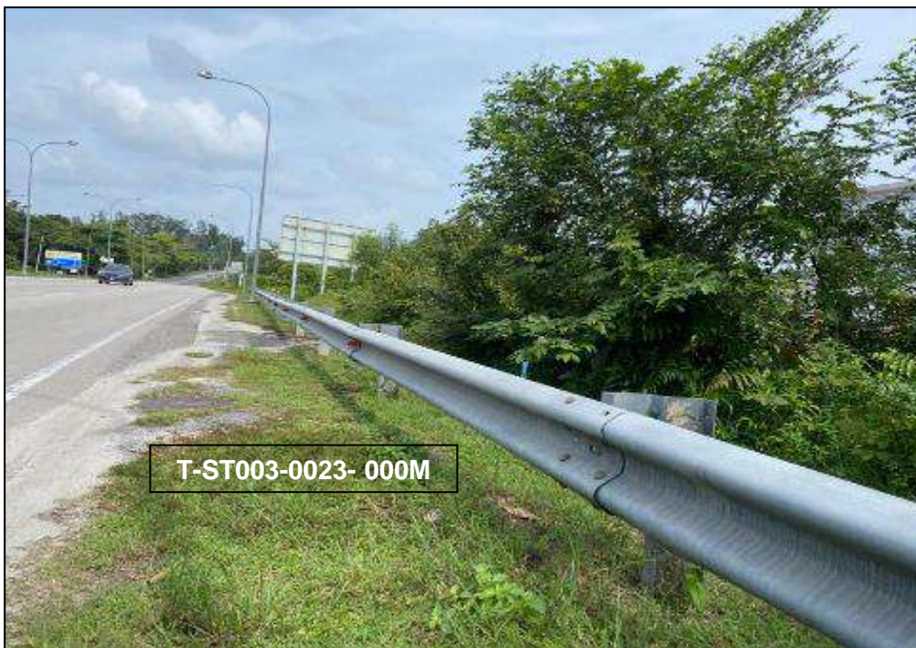
LOCATION AT JALAN KUALA TERENGGANU
