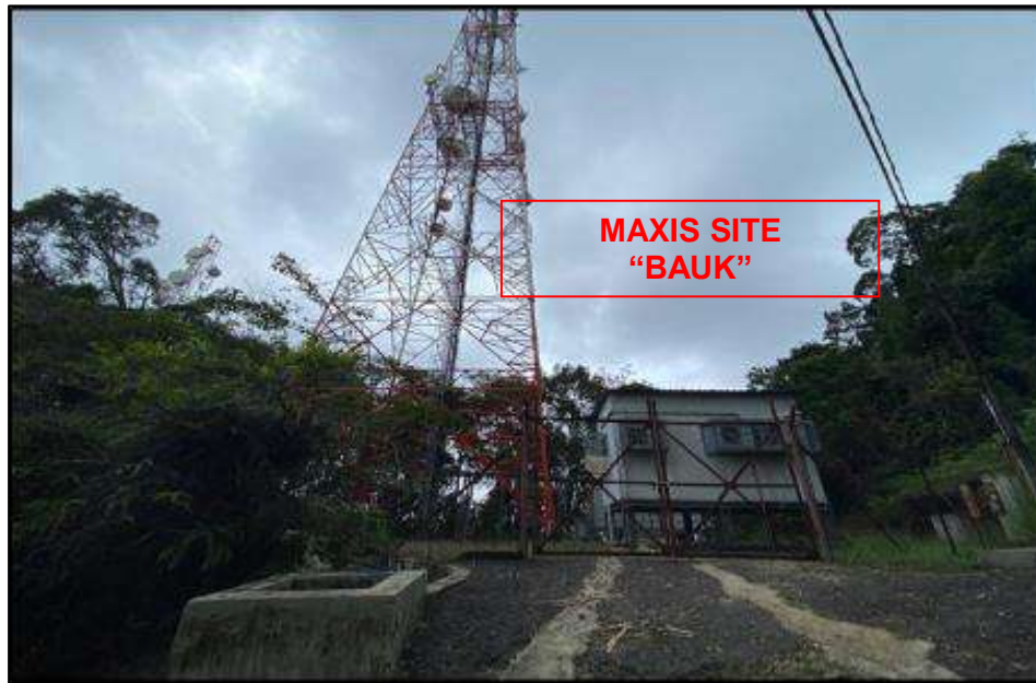
LOCATION AT SITE BAUK
