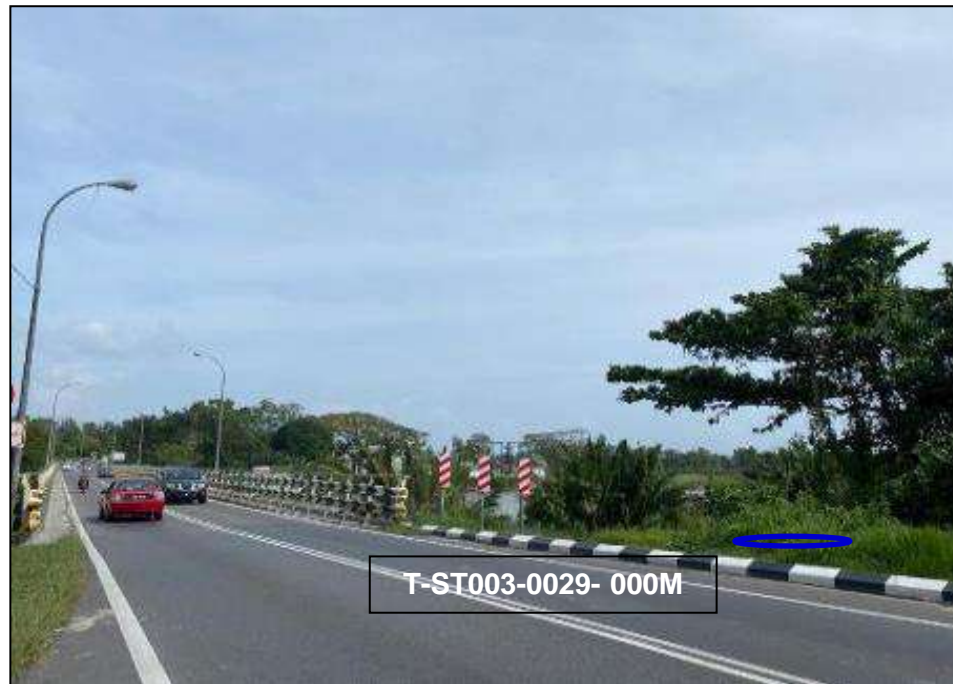
LOCATION AT JALAN KUALA TERENGGANU
