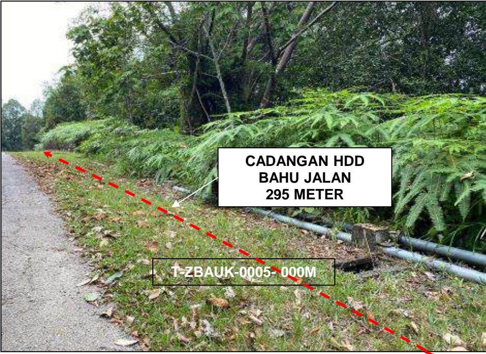
LOCATION AT SITE BAUK
