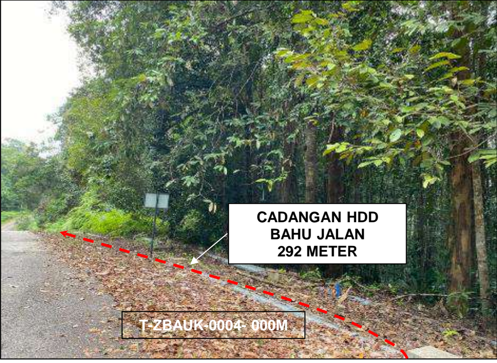
LOCATION AT SITE BAUK
