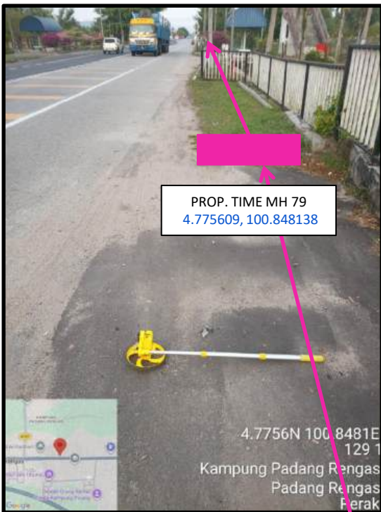
Proposed HDD 1 Way and Pulling Cable 144C from Prop. TIME MH79 to Prop. TIME MH80 at Kampung Padang Rengas
