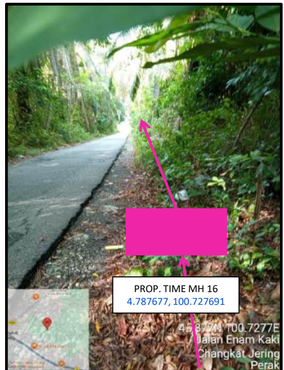
Proposed HDD 1 Way and Pulling Cable 144C from Prop. TIME MH16 to Prop. TIME MH17 at Jalan Enam Kaki
