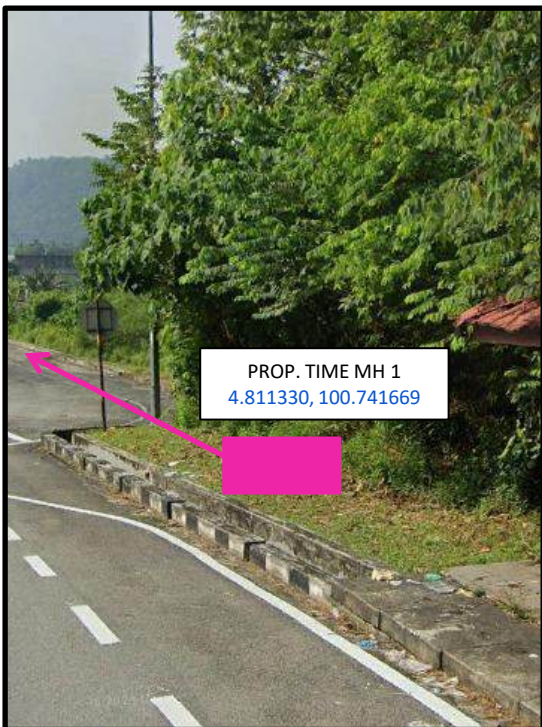
Proposed HDD 1 Way and Pulling Cable 144C from Prop. TIME MH01 to Prop. TIME MH02 at Taman Kuning Sari
