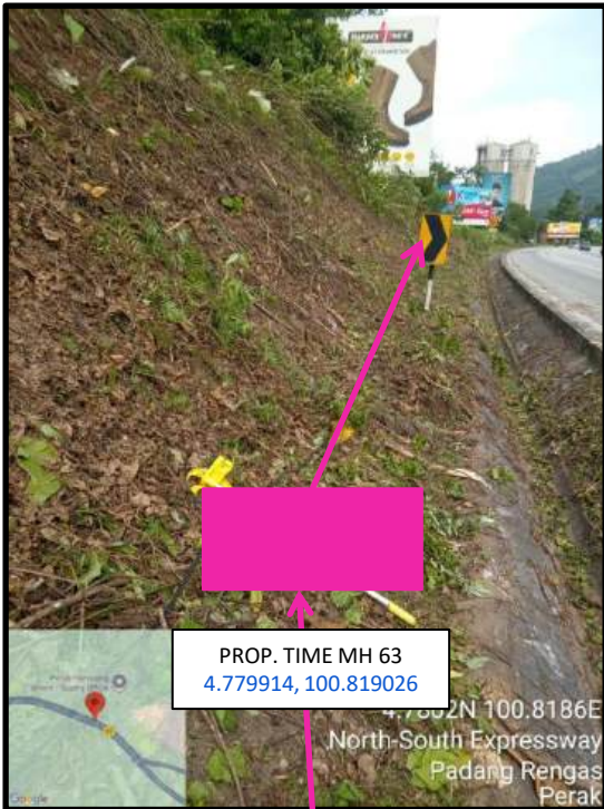
Proposed HDD 1 Way and Pulling Cable 144C from Prop. TIME MH63 to Prop. TIME MH64 at beside the highway
