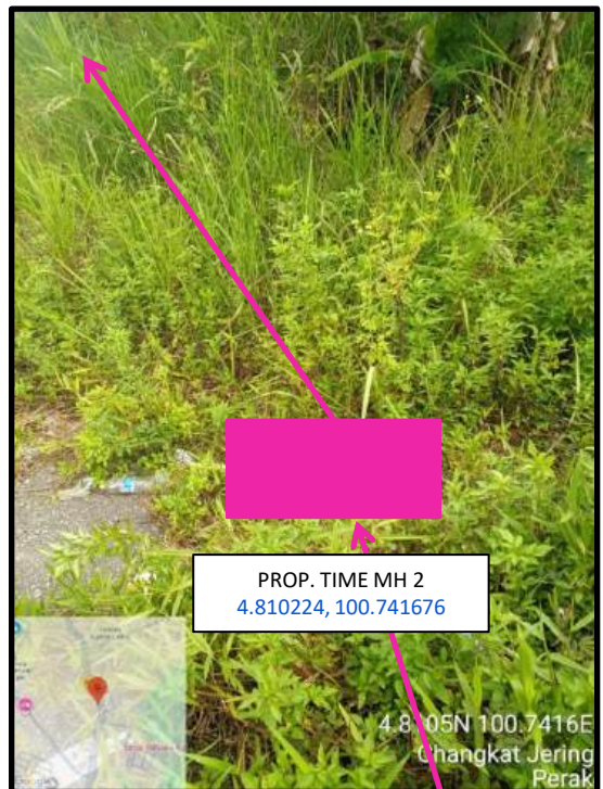
Proposed HDD 1 Way and Pulling Cable 144C from Prop. TIME MH02 to Prop. TIME MH03 at Taman Kuning Sari
