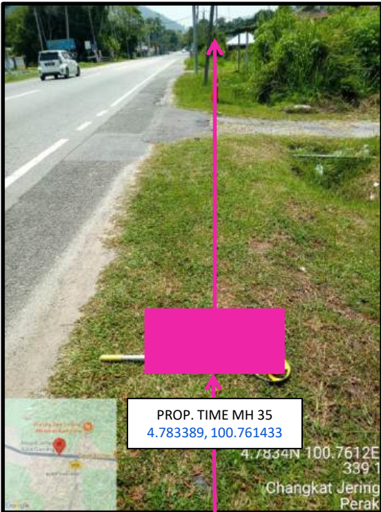
Proposed HDD 1 Way and Pulling Cable 144C from Prop. TIME MH35 to Prop. TIME MH36 at Bukit Gantang
