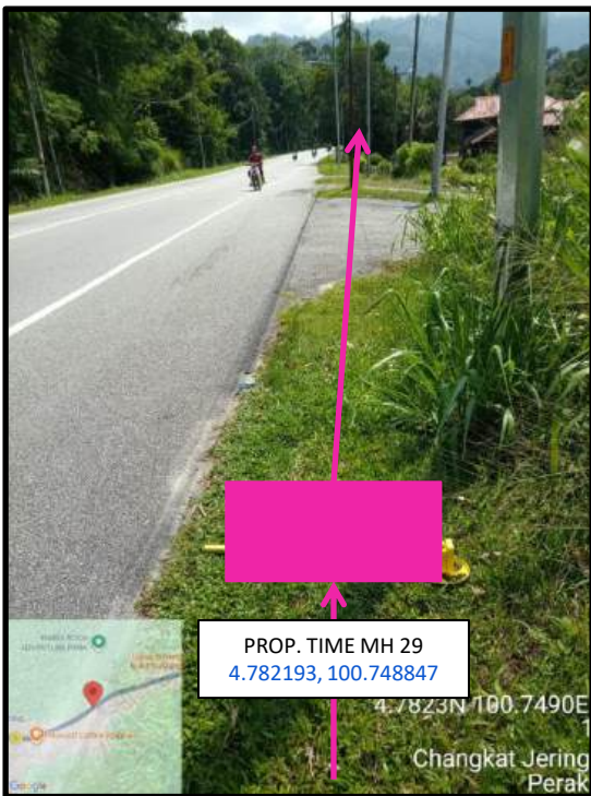
Proposed HDD 1 Way and Pulling Cable 144C from Prop. TIME MH29 to Prop. TIME MH30 at Changkat Jering
