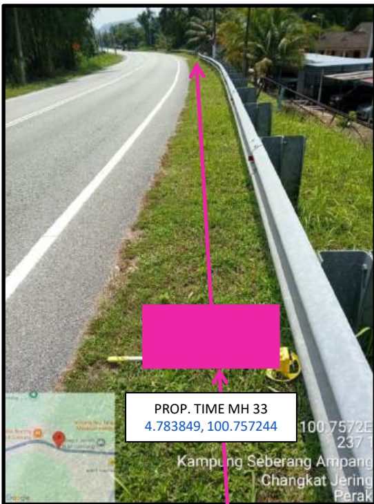
Proposed HDD 1 Way and Pulling Cable 144C from Prop. TIME MH33 to Prop. TIME MH34 at Bukit Gantang
