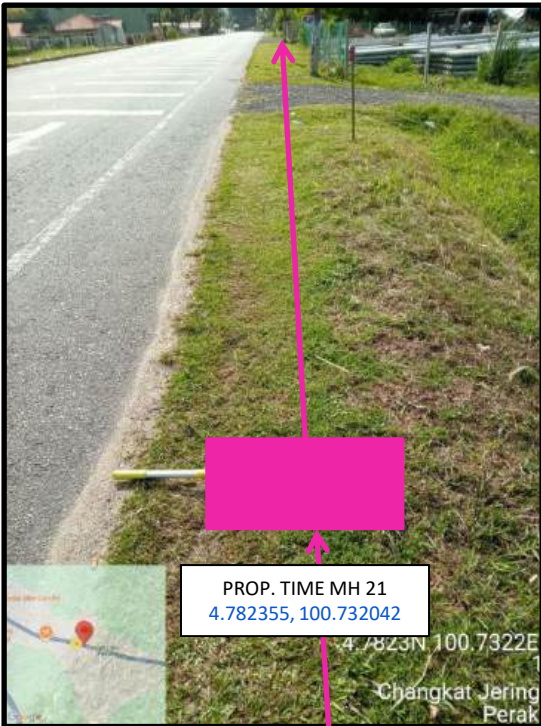
Proposed HDD 1 Way and Pulling Cable 144C from Prop. TIME MH21 to Prop. TIME MH22 at Jalan Enam Kaki
