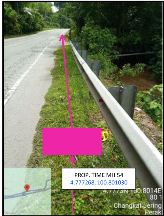
Proposed HDD 1 Way and Pulling Cable 144C from Prop. TIME MH54 to Prop. TIME MH55 at beside the highway
