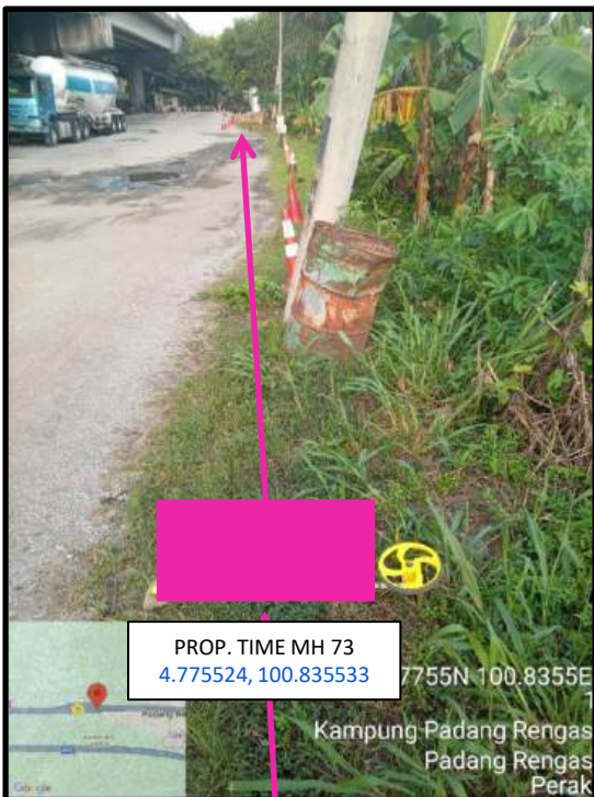
Proposed HDD 1 Way and Pulling Cable 144C from Prop. TIME MH73 to Prop. TIME MH74 at Kampung Padang Rengas
