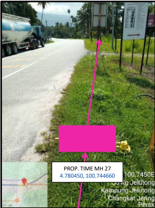
Proposed HDD 1 Way and Pulling Cable 144C from Prop. TIME MH27 to Prop. TIME MH28 at Jalan Enam Kaki
