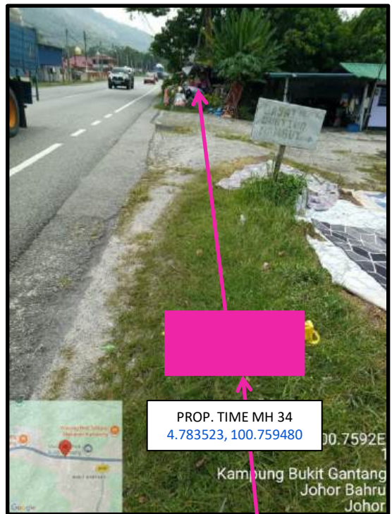
Proposed HDD 1 Way and Pulling Cable 144C from Prop. TIME MH34 to Prop. TIME MH35 at Bukit Gantang
