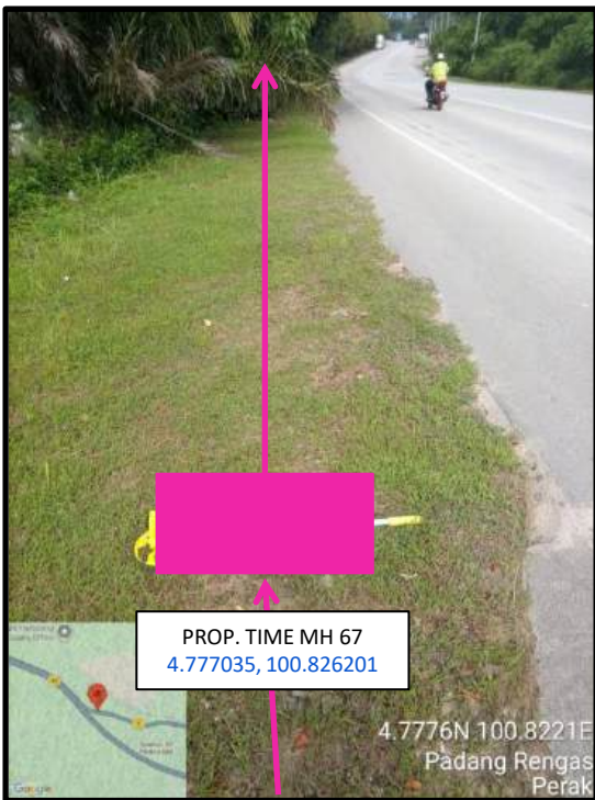
Proposed HDD 1 Way and Pulling Cable 144C from Prop. TIME MH67 to Prop. TIME MH68 at Jalan Abdul Shukor
