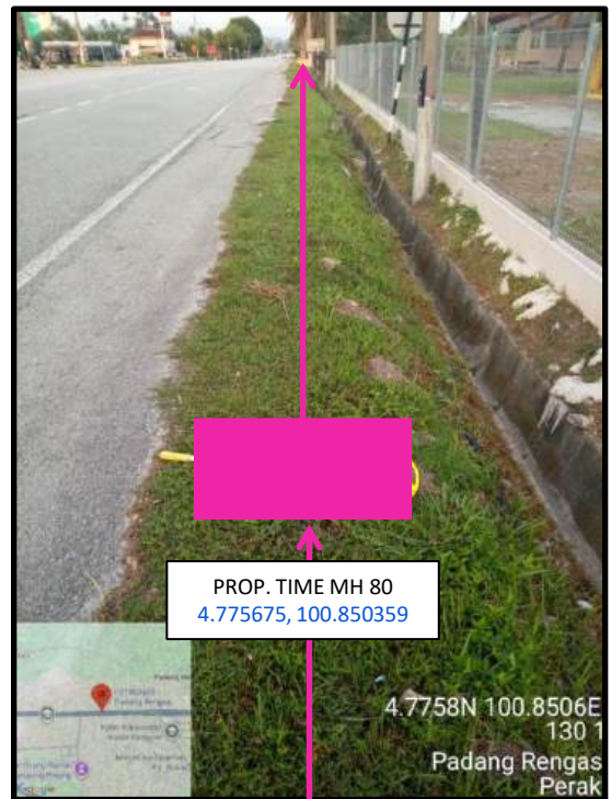
Proposed HDD 1 Way and Pulling Cable 144C from Prop. TIME MH80 to Prop. TIME MH81 at Kampung Padang Rengas
