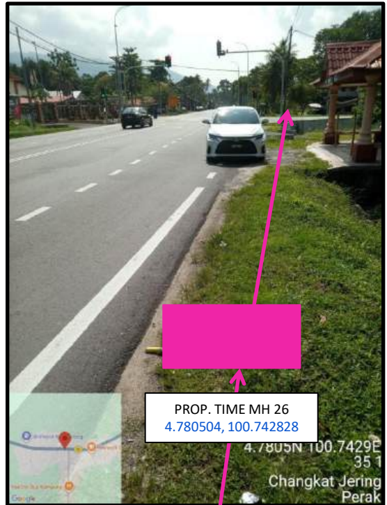
Proposed HDD 1 Way and Pulling Cable 144C from Prop. TIME MH26 to Prop. TIME MH27 at Jalan Enam Kaki
