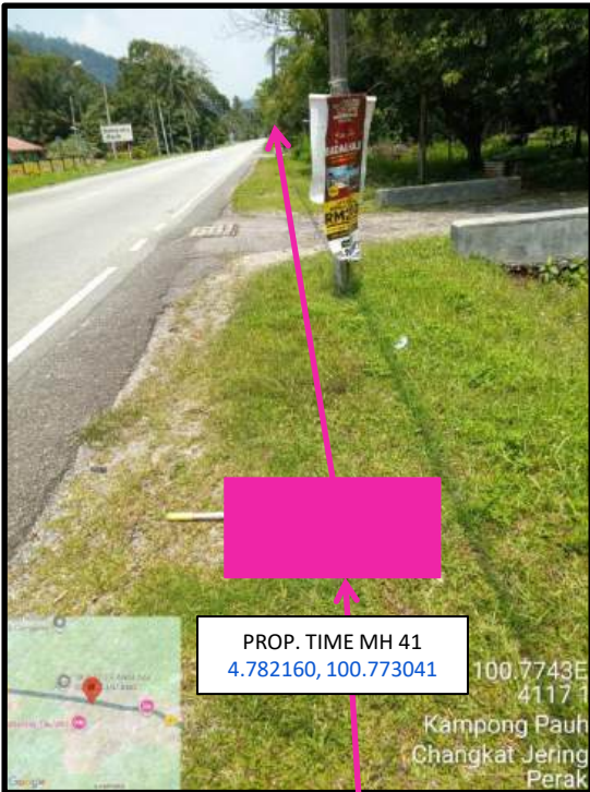
Proposed HDD 1 Way and Pulling Cable 144C from Prop. TIME MH41 to Prop. TIME MH42 at Kampong Pauh
