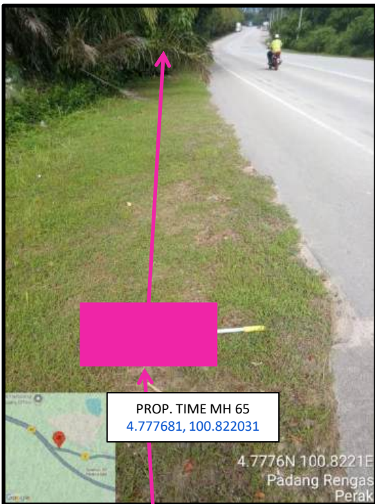
Proposed HDD 1 Way and Pulling Cable 144C from Prop. TIME MH65 to Prop. TIME MH66 at beside the highway
