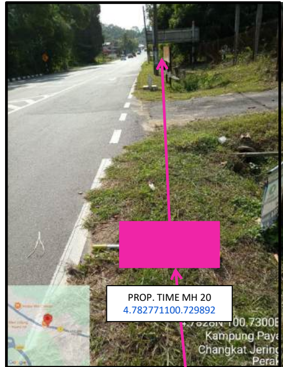
Proposed HDD 1 Way and Pulling Cable 144C from Prop. TIME MH20 to Prop. TIME MH21 at Kampung Paya
