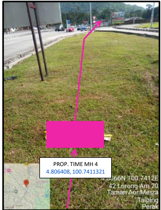
Proposed HDD 1 Way and Pulling Cable 144C from Prop. TIME MH04 to Prop. TIME MH05 at Taman Aor Mesra
