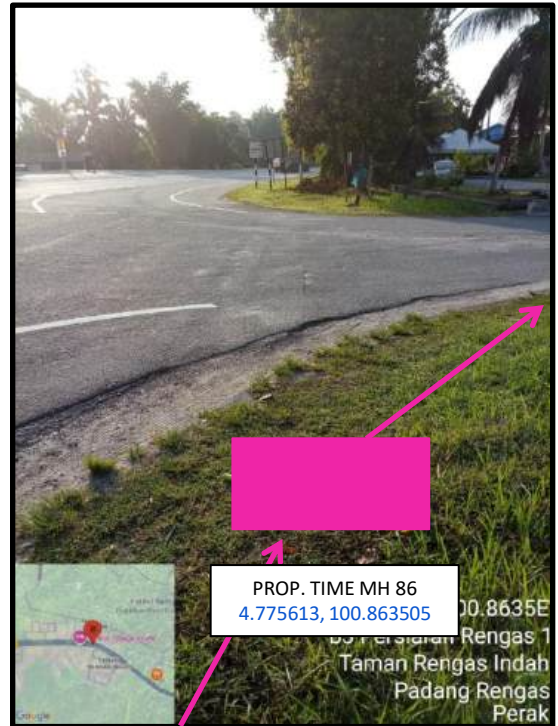
Proposed HDD 1 Way and Pulling Cable 144C from Prop. TIME MH86 to Prop. TIME MH87 at Kampung Padang Rengas
