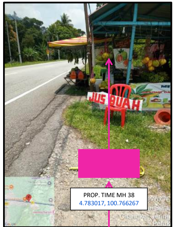
Proposed HDD 1 Way and Pulling Cable 144C from Prop. TIME MH38 to Prop. TIME MH39 at Bukit Gantang
