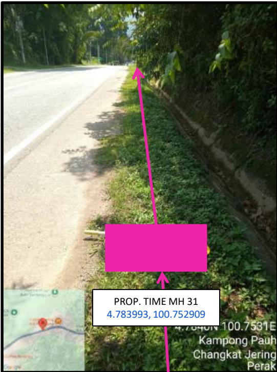
Proposed HDD 1 Way and Pulling Cable 144C from Prop. TIME MH31 to Prop. TIME MH32 at Kampong Pauh
