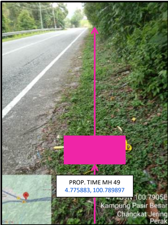
Proposed HDD 1 Way and Pulling Cable 144C from Prop. TIME MH49 to Prop. TIME MH50 at Kampung Pasir Besar
