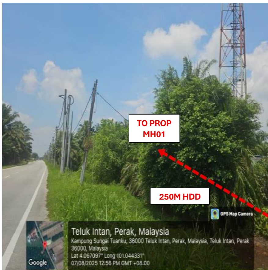
PICTURE 2 : HDD 250METER TO PROPOSE MH01
