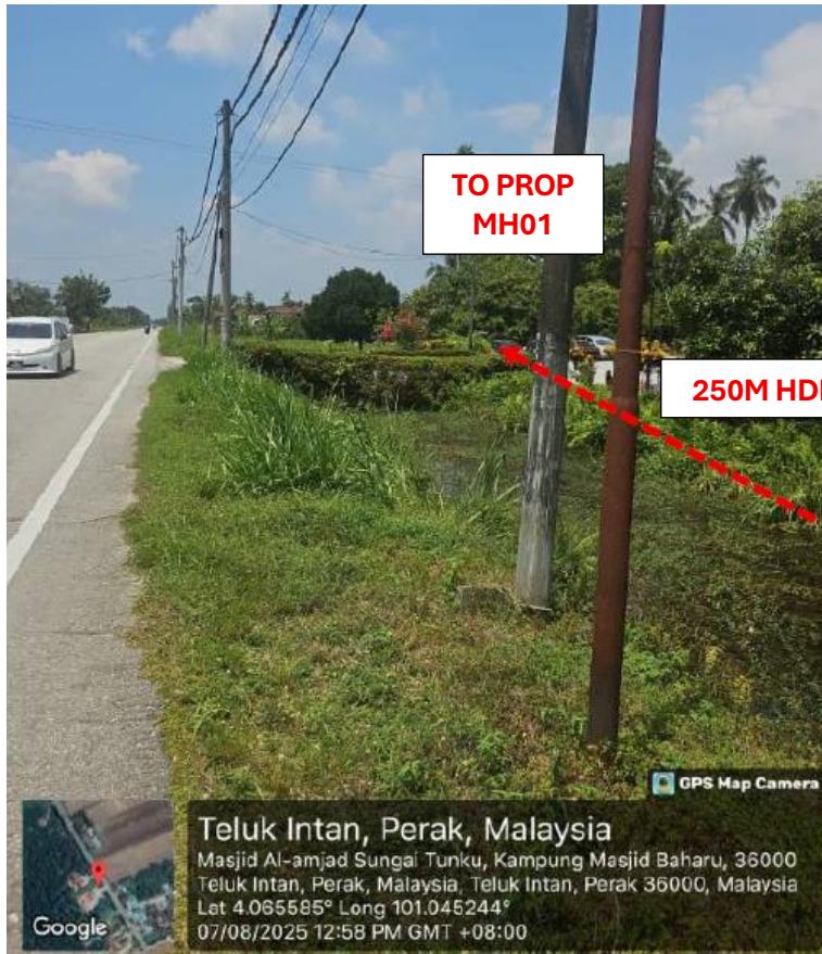
PICTURE 4 : HDD 250METER TO PROPOSE MH01
