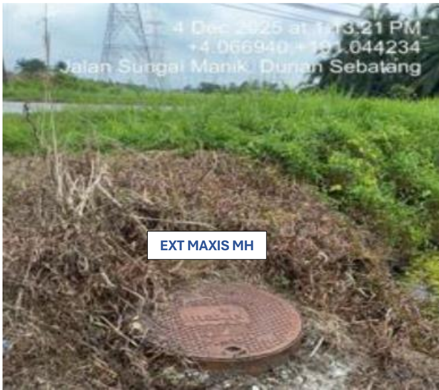
PICTURE 1 : EXISTING MAXIS MANHOLE
