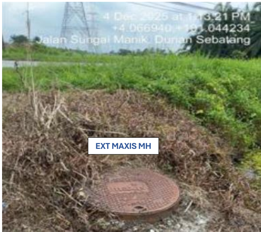
PICTURE 1 : EXISTING MAXIS MANHOLE
