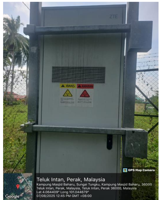
Picture 7: USING PN12.5 CONDUIT TOWARDS CABINET T5
