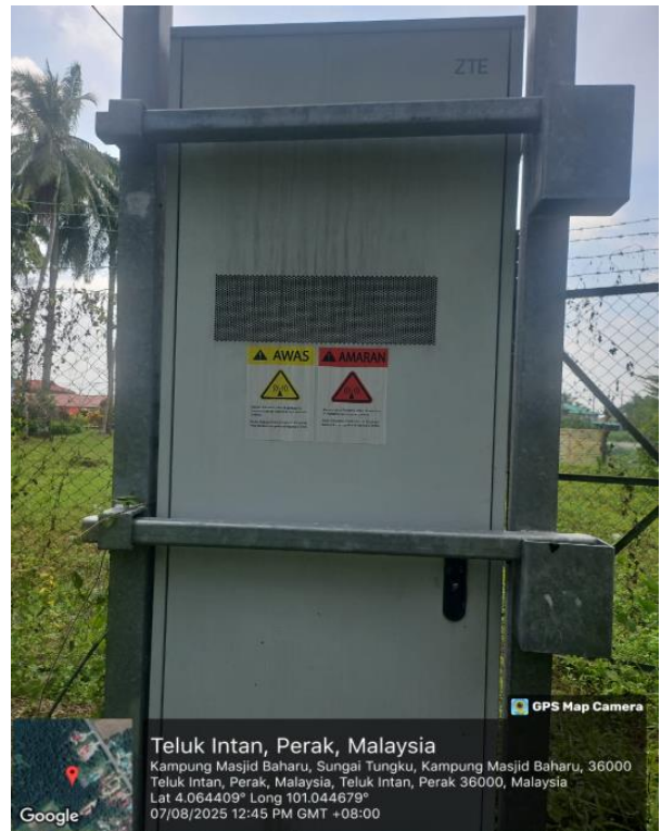
Picture 7: USING PN12.5 CONDUIT TOWARDS CABINET T5
