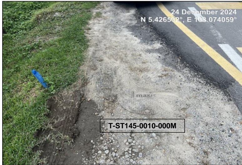
LOCATION AT JALAN (T145)
