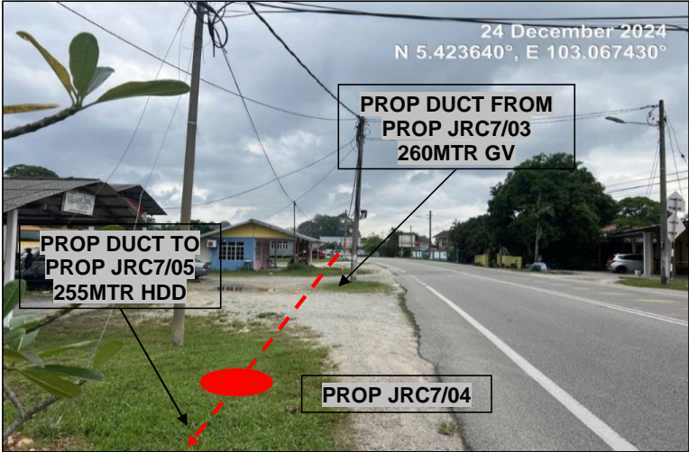
LOCATION AT JALAN KG PADANG MARAS- KG TELIPOT (T148)
