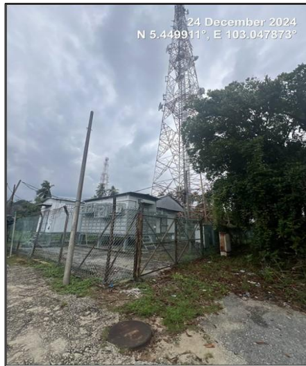
LOCATION AT MAXIS SITE "RAKI"
