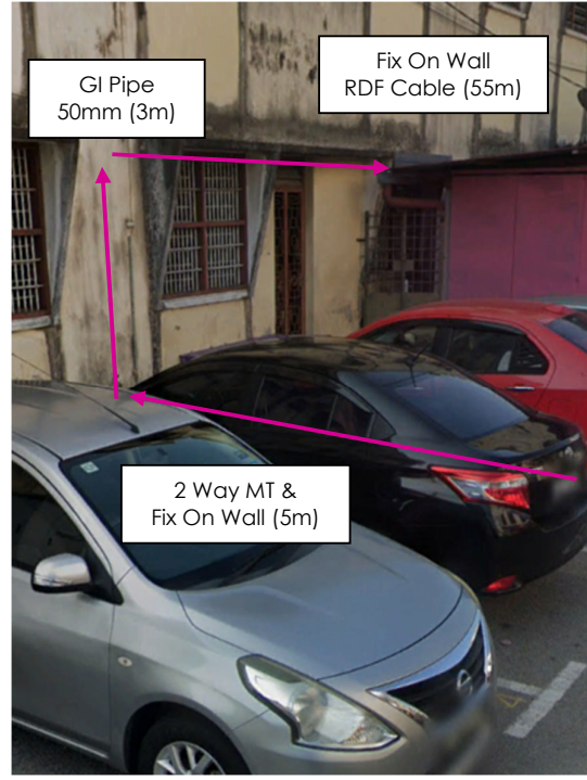
Proposed GI Pipe & RDF Cable at Jalan Sirat
