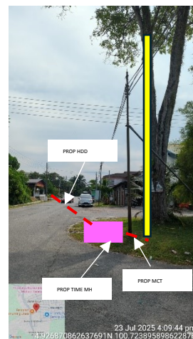
PROP POLE, HDD , TIME MH AT JALAN TAMAN LELA
