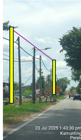
PROP POLE AT JALAN BUKIT JANA INDAH 6
