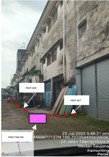
PROP HDD , TIME MH and MCT AT BACKLANE JALAN TAIPING UTARA
