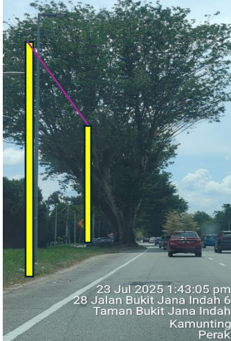
PROP POLE AT JALAN BUKIT JANA INDAH 6
