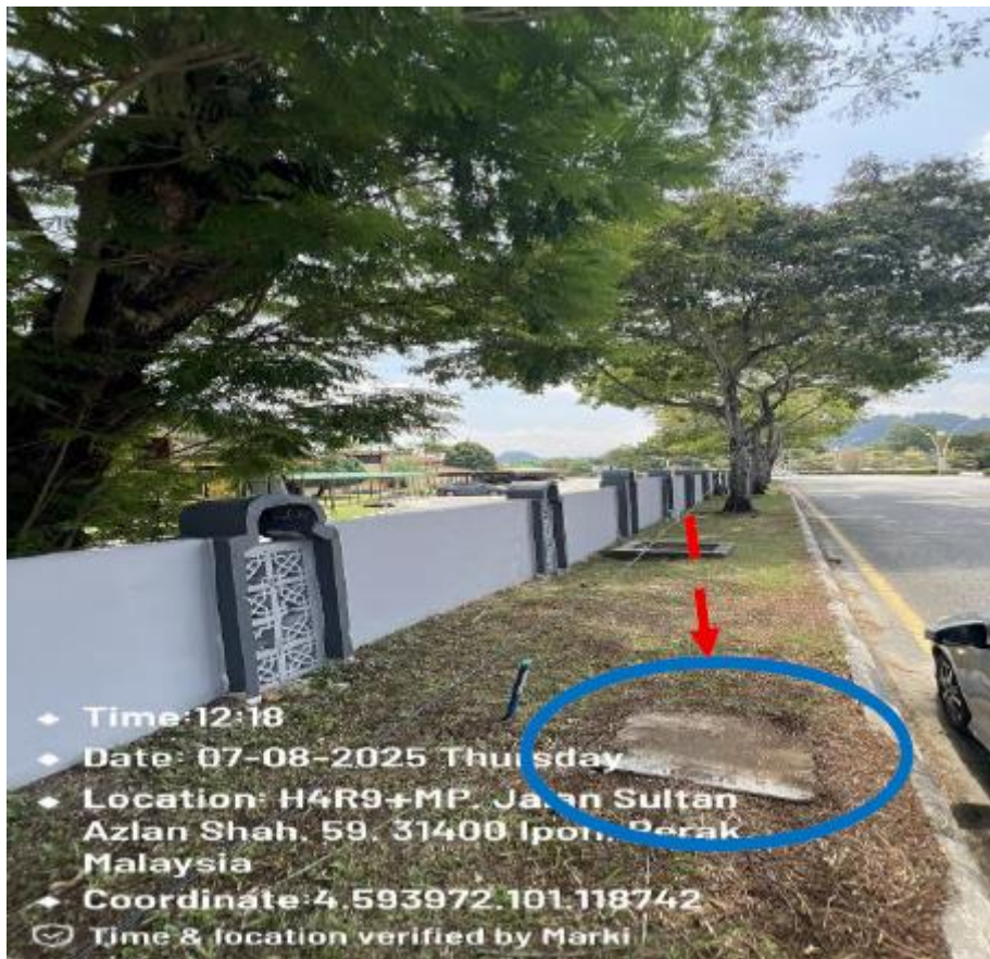
PICTURE 1 : EXISTING MAXIS MANHOLE
