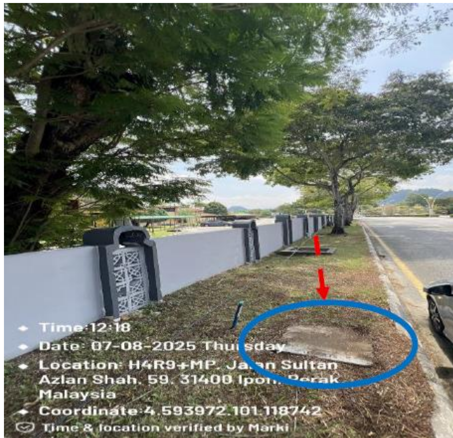
PICTURE 1 : EXISTING MAXIS MANHOLE
