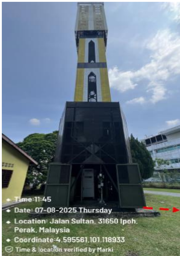
PICTURE 8 : 50M MICROTRENCHING TO UM T5 FROM MH01
