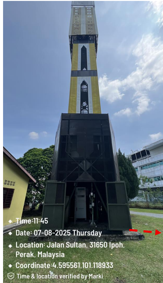
PICTURE 2: PROPOSE MICRO TRENCHING
