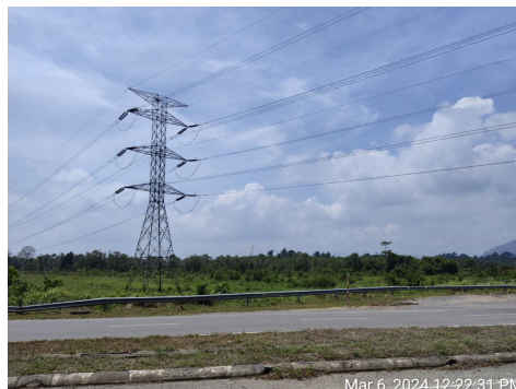
TNB Pylon – Open Cut (4.621333° 103.414018°)
