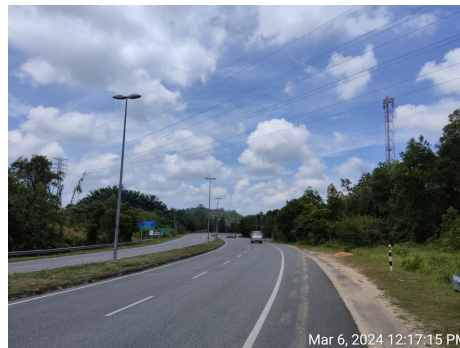
TNB Pylon – Open Cut (4.621303° 103.376168°)
