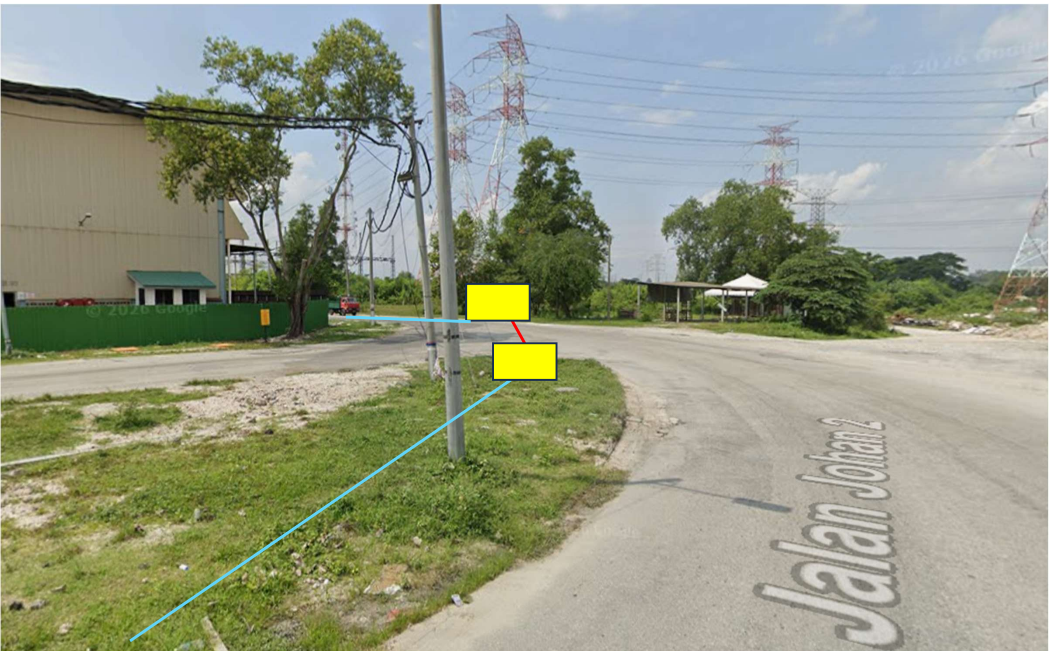
JALAN JOHAN 2 OPEN CUT & HDD
