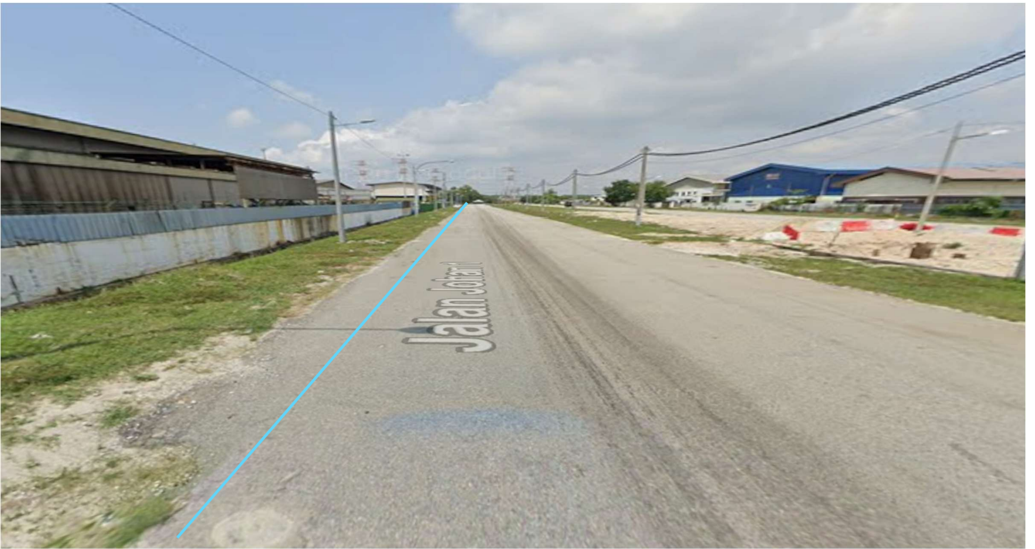
JALAN JOHAN 2 OPEN CUT
