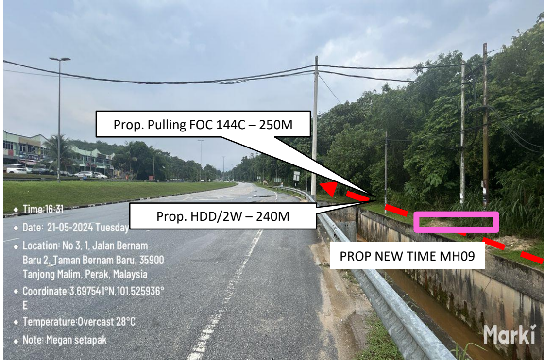
Proposed HDD/2W (250M) and pulling FOC 144C (260M) from Prop New TIME MH09 to Prop New TIME MH10
