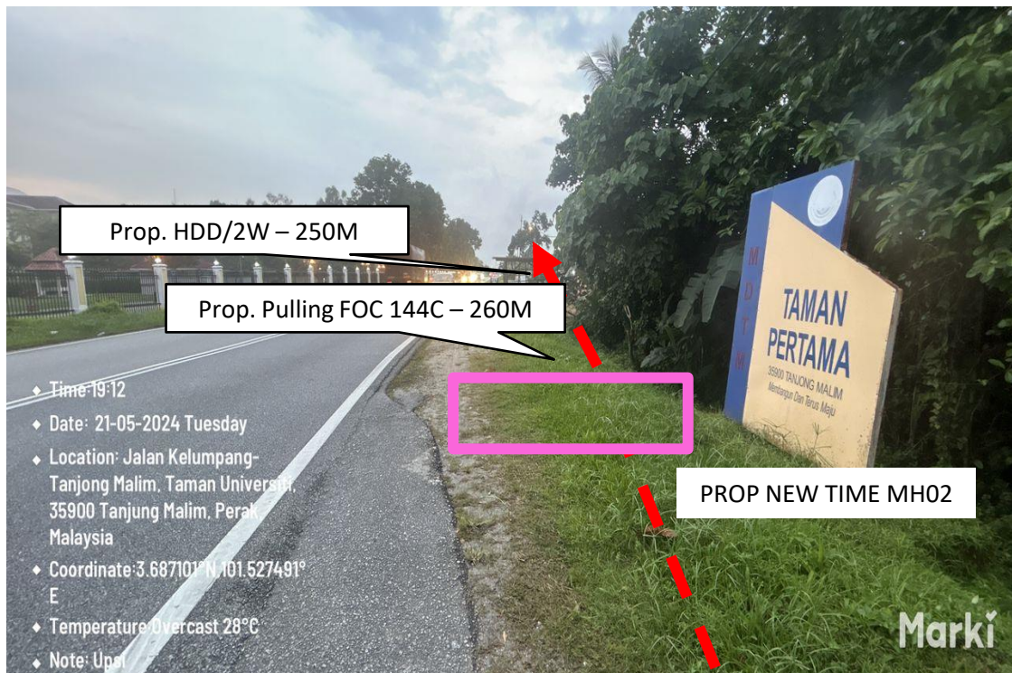
Proposed HDD/2W (250M) and pulling FOC 144C (260M) from Prop New TIME MH02 to Prop New TIME MH03
