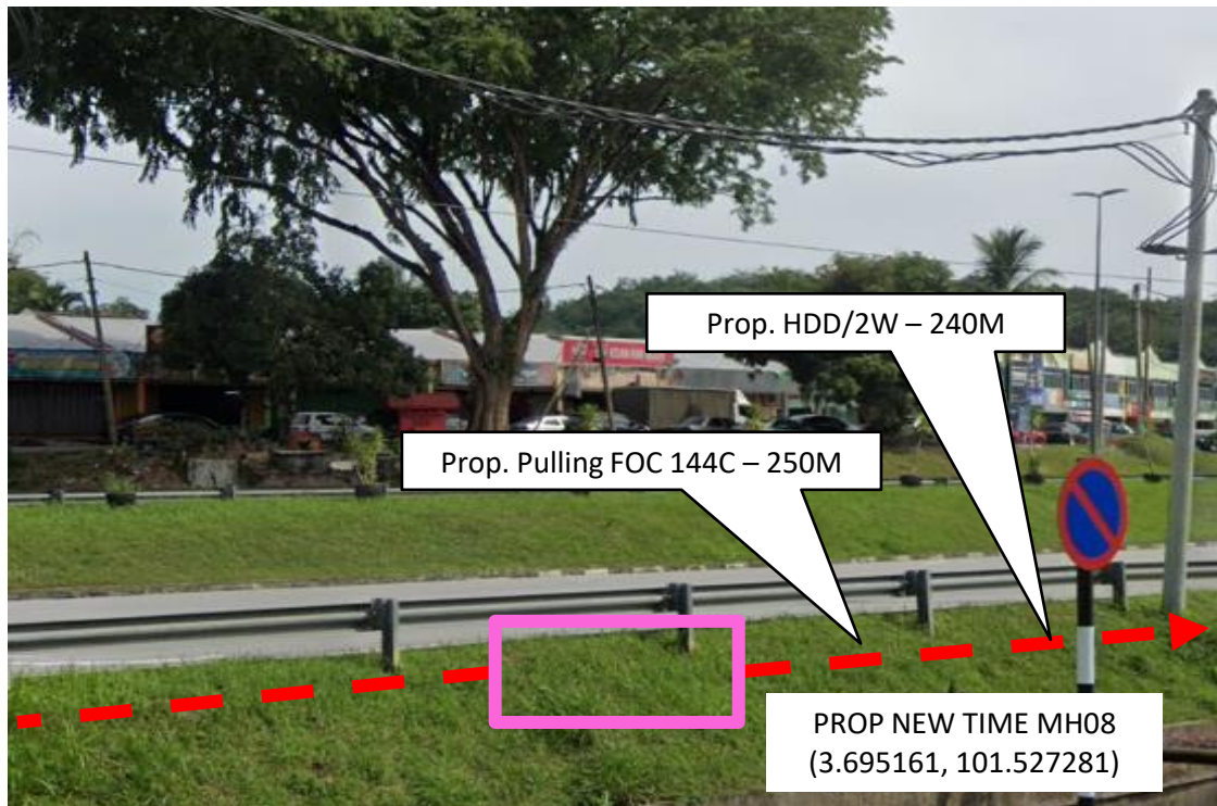
Proposed HDD/2W (250M) and pulling FOC 144C (260M) from Prop New TIME MH08 to Prop New TIME MH09
