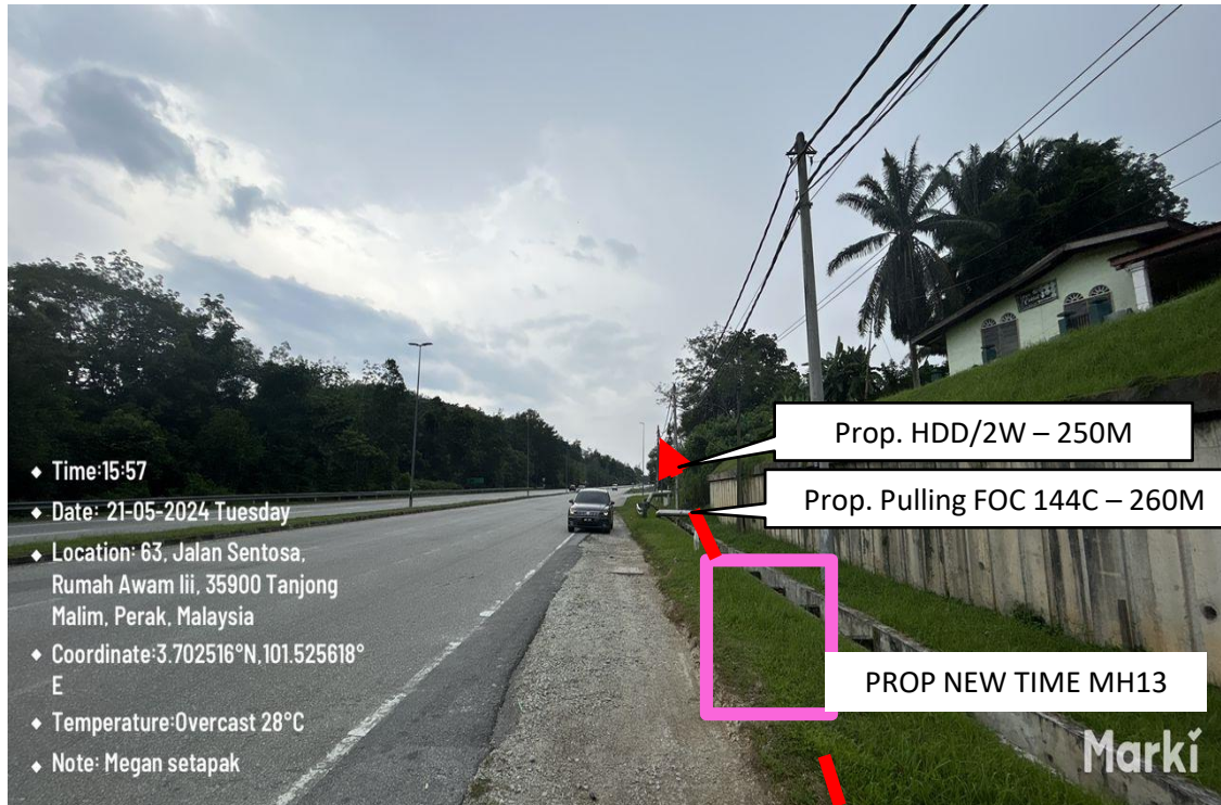
Proposed HDD/2W (250M) and pulling FOC 144C (260M) from Prop New TIME MH13 to Prop New TIME MH14
