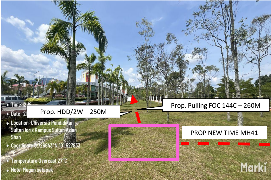
Proposed HDD/2W (250M) and pulling FOC 144C (260M) from Prop New TIME MH41 to EXT BMH01
