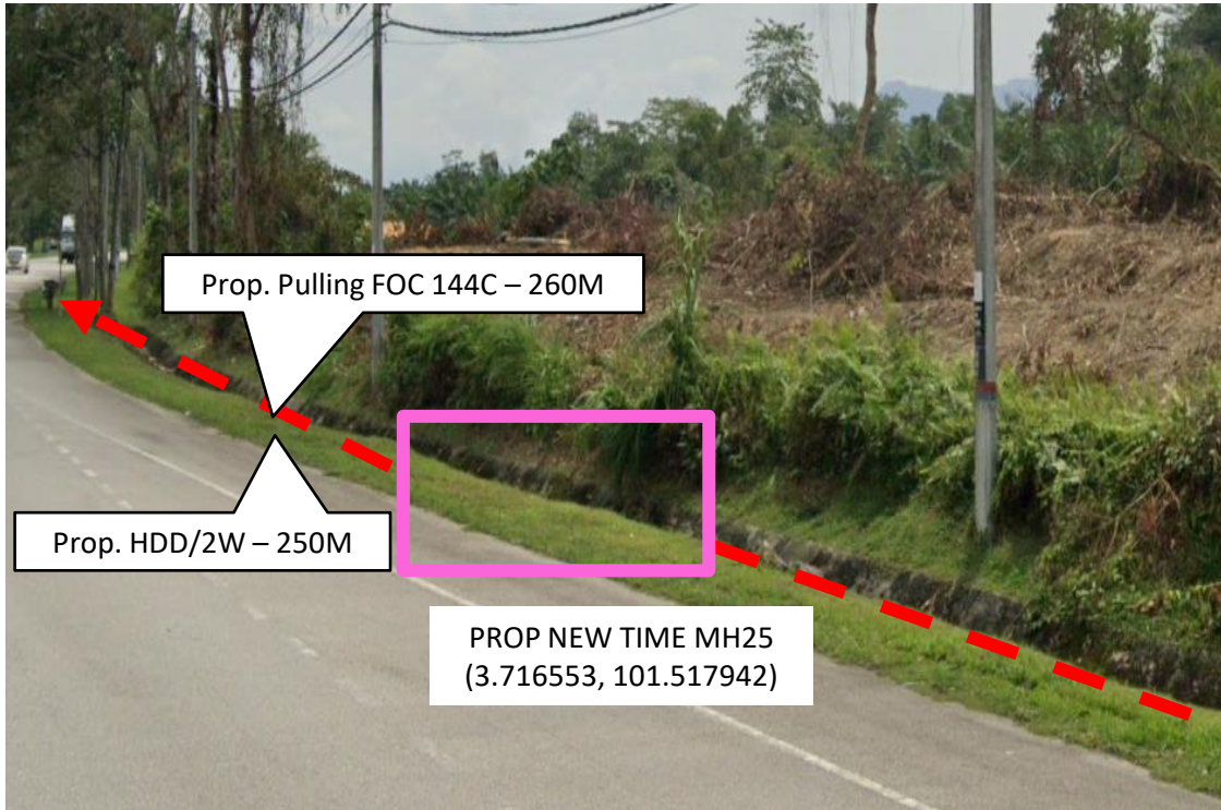
Proposed HDD/2W (250M) and pulling FOC 144C (260M) from Prop New TIME MH25 to Prop New TIME MH26
