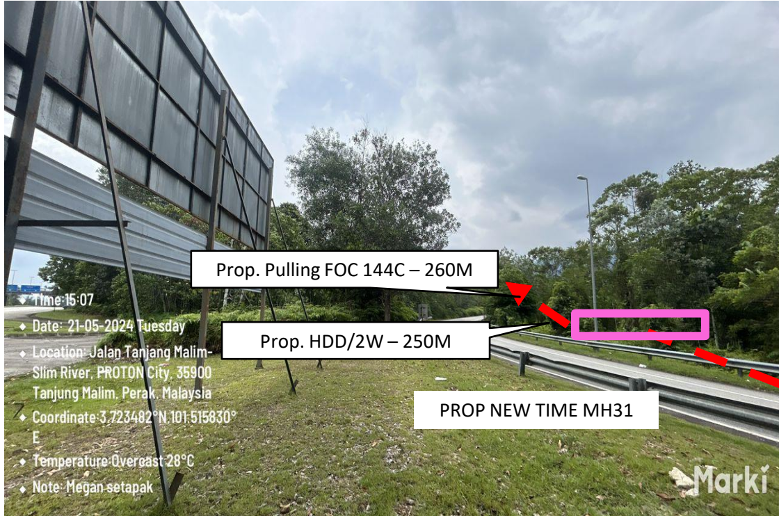
Proposed HDD/2W (250M) and pulling FOC 144C (260M) from Prop New TIME MH31 to Prop New TIME MH32
