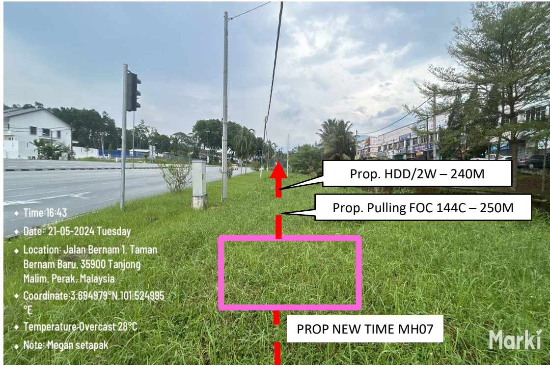
Proposed HDD/2W (250M) and pulling FOC 144C (260M) from Prop New TIME MH07 to Prop New TIME MH08
