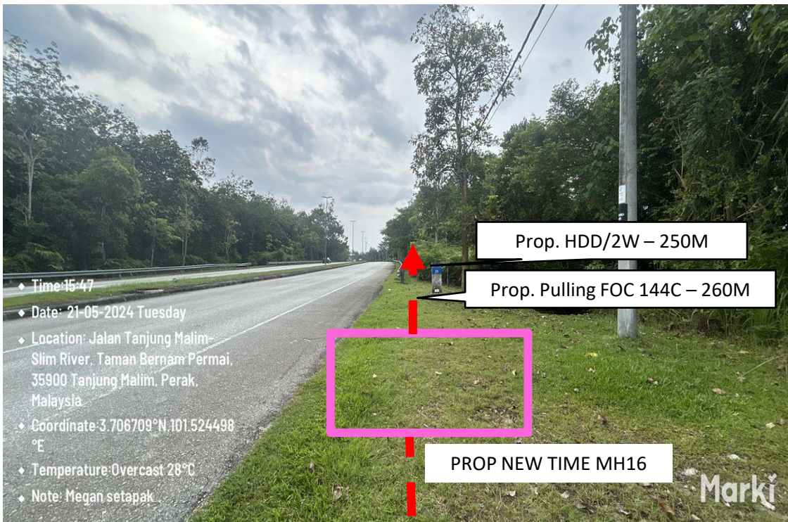
Proposed HDD/2W (250M) and pulling FOC 144C (260M) from Prop New TIME MH16 to Prop New TIME MH17
