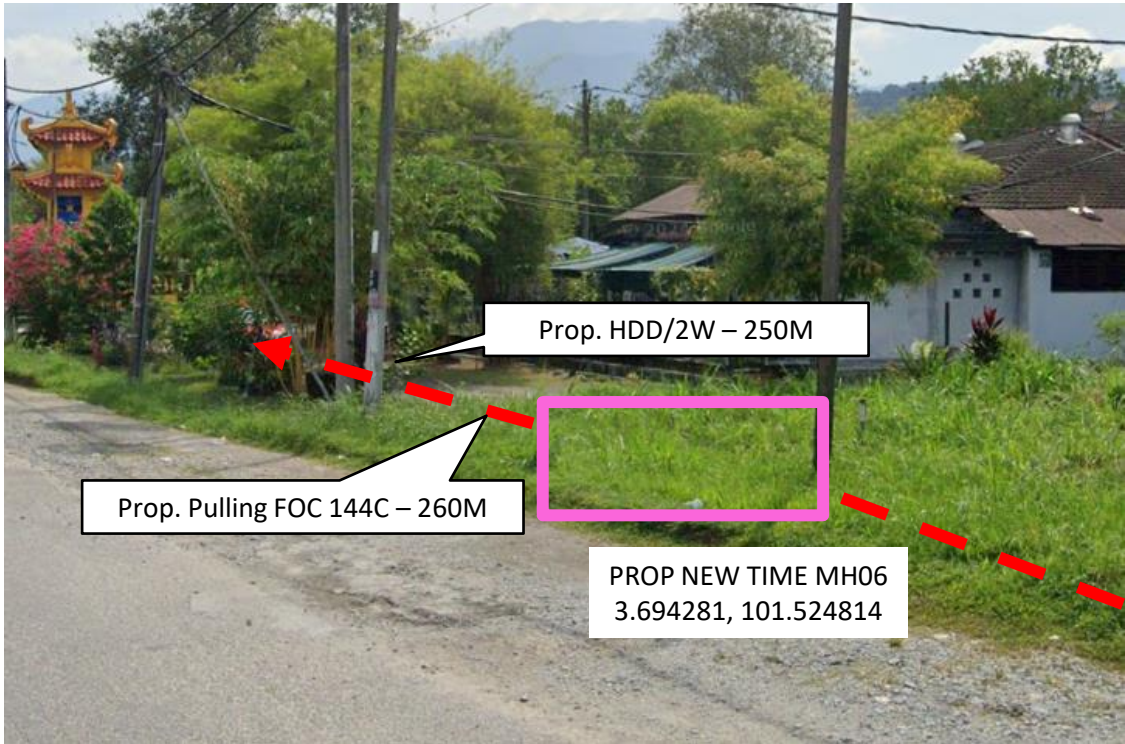
Proposed HDD/2W (250M) and pulling FOC 144C (260M) from Prop New TIME MH06 to Prop New TIME MH07
