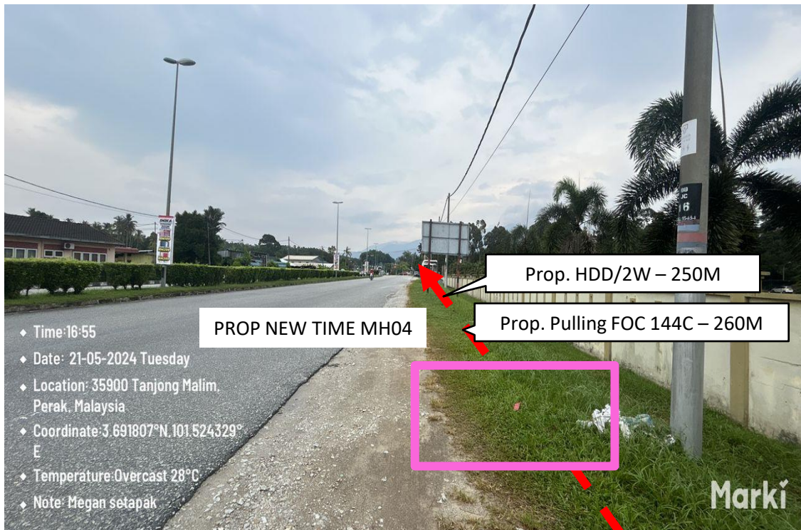
Proposed HDD/2W (250M) and pulling FOC 144C (260M) from Prop New TIME MH04 to Prop New TIME MH05
