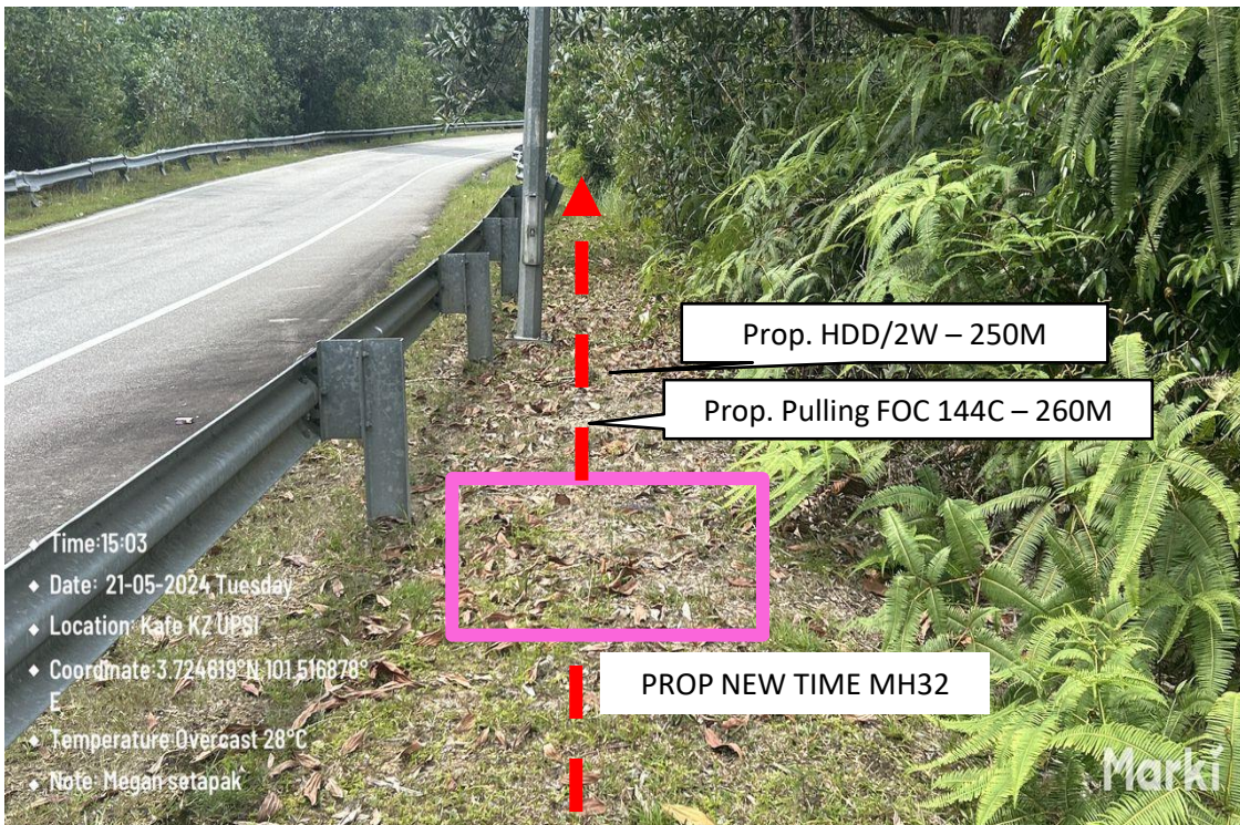
Proposed HDD/2W (250M) and pulling FOC 144C (260M) from Prop New TIME MH32 to Prop New TIME MH33
