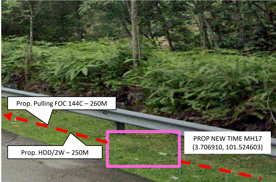
Proposed HDD/2W (250M) and pulling FOC 144C (260M) from Prop New TIME MH17 to Prop New TIME MH18
