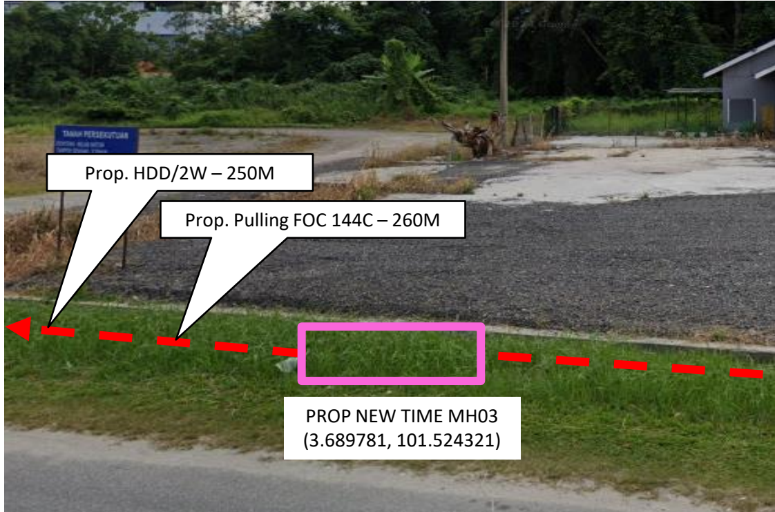
Proposed HDD/2W (250M) and pulling FOC 144C (260M) from Prop New TIME MH03 to Prop New TIME MH04
