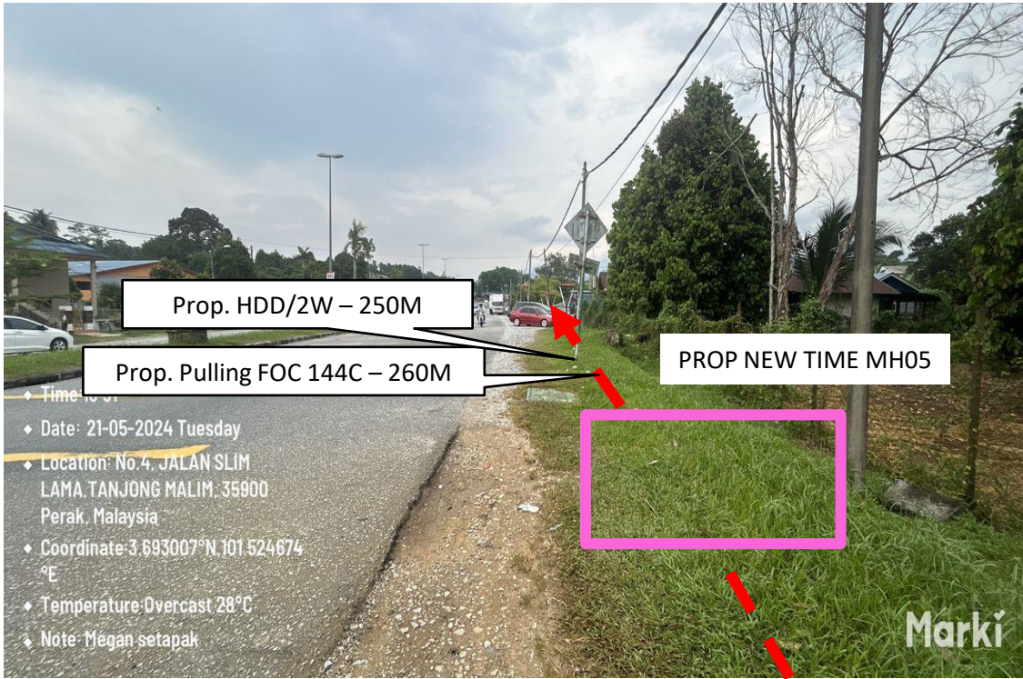
Proposed HDD/2W (250M) and pulling FOC 144C (260M) from Prop New TIME MH05 to Prop New TIME MH06
