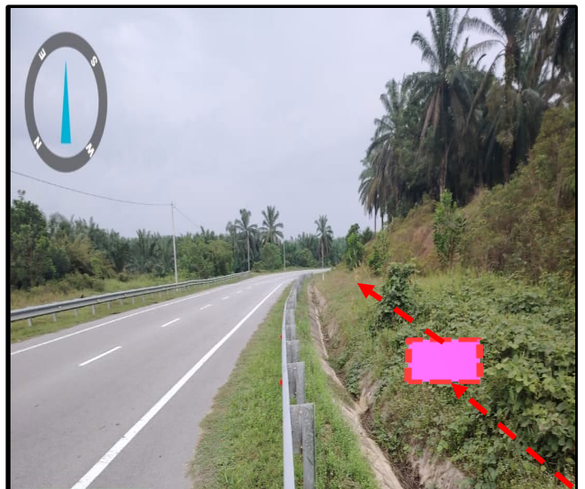
Prop New TIME MH 35 (Jln Kubu Gajah-Taiping)( 5.111094° , 100.716663° )
