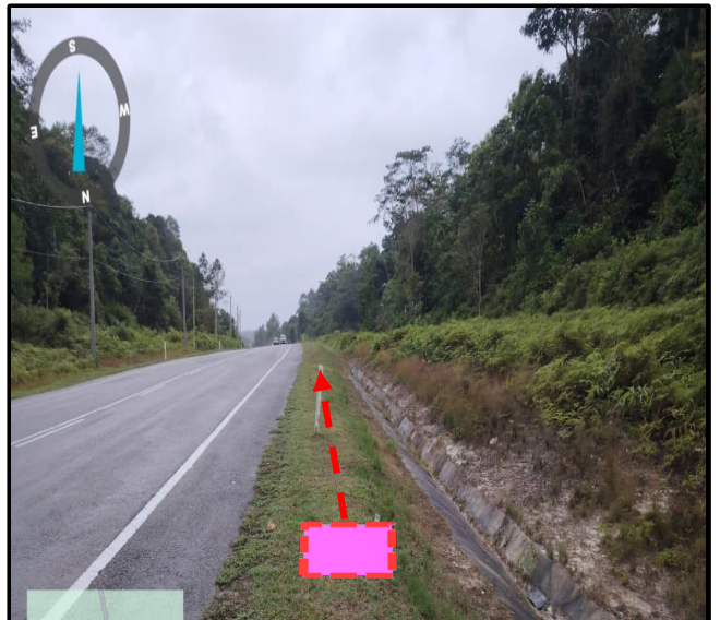
Prop New TIME MH51 (Jln Kubu Gajah-Taiping)( 5.075503° , 100.720095° )
