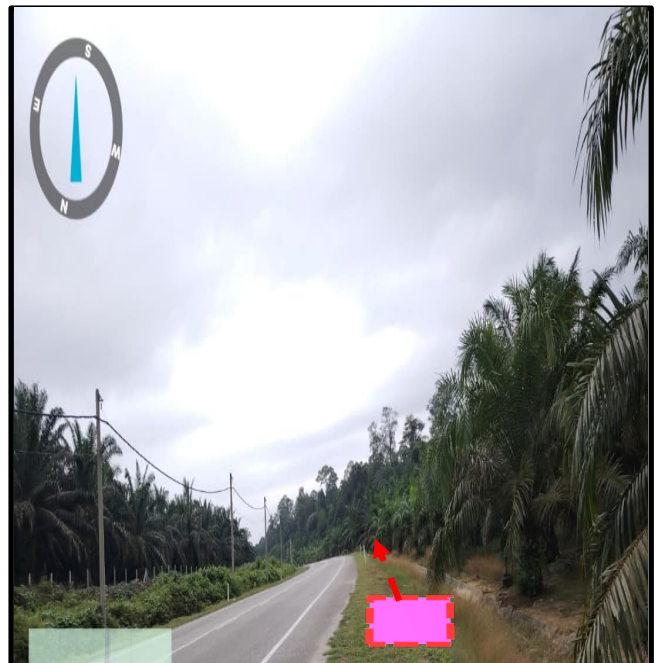
Prop New TIME MH 47 (Jln Kubu Gajah-Taiping)(5.084441°, 100.719728°)
