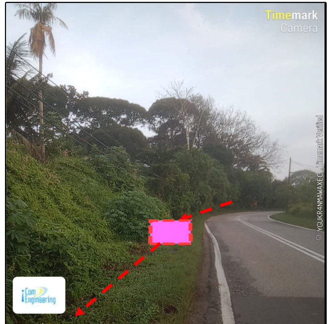
Prop New TIME MH 85 (Jln Kubu Gajah-Taiping)( 5.005989° , 100.733152° )
