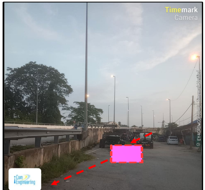
Prop New TIME MH 83 (Jln Kubu Gajah-Taiping)( 5.009828° , 100.730843° )
