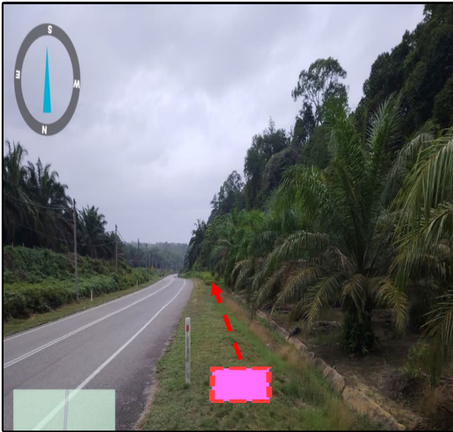
Prop New TIME MH 48 (Jln Kubu Gajah-Taiping)( 5.082261° , 100.720261° )
