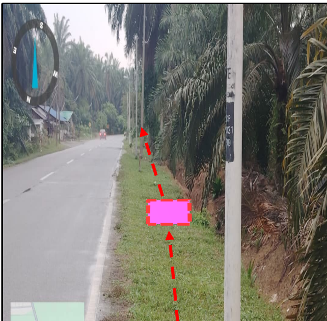
Prop New TIME MH 78 (Jln Kubu Gajah-Taiping)( 5.017560° , 100.732221° )
