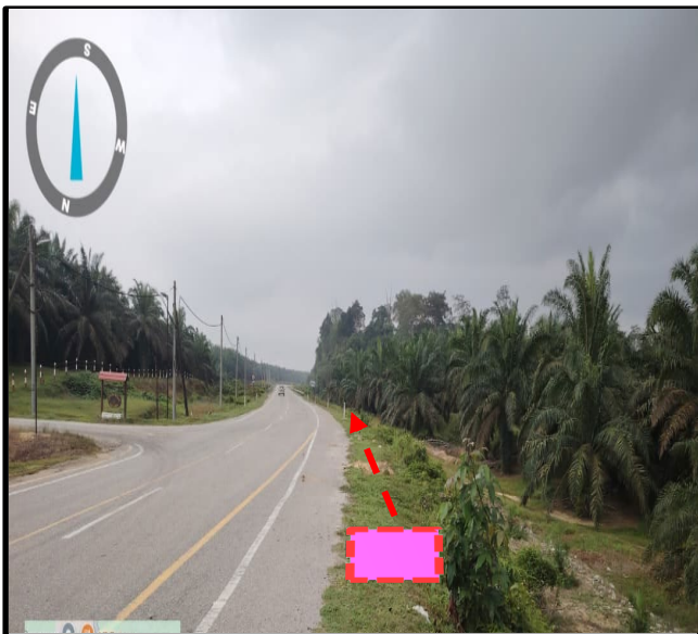
Prop New TIME MH 42 (Jln Kubu Gajah-Taiping)( 5.095618°, 100.719326° )
