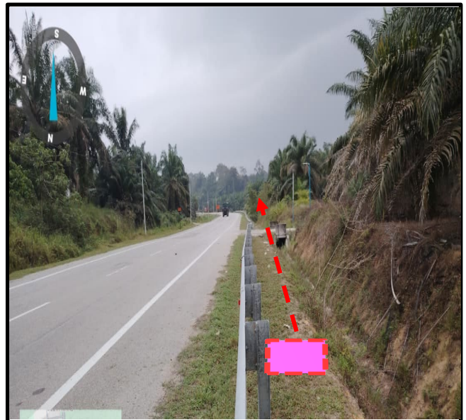
Prop New TIME MH 41 (Jln Kubu Gajah-Taiping) ( 5.097762°, 100.718636° )
