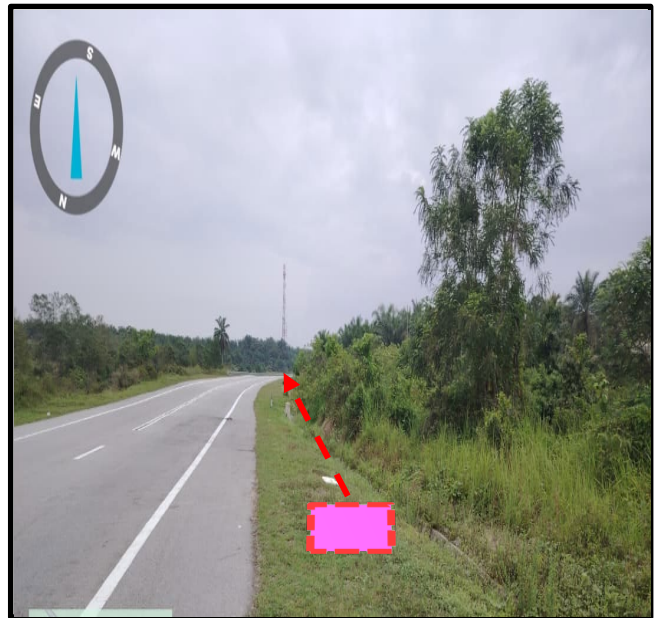
Prop New TIME MH 37 (Jln Kubu Gajah-Taiping)(5.106637°, 100.717440°)
