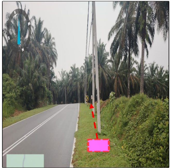
Prop New TIME MH 73 (Jln Kubu Gajah-Taiping)( 5.027828° , 100.728874° )
