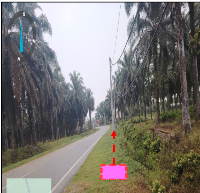
Prop New TIME MH 74 (Jln Kubu Gajah-Taiping)( 5.025777° , 100.729849° )
