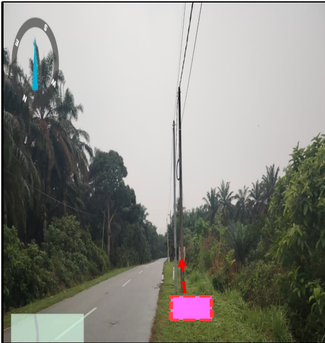
Prop New TIME MH 76 (Jln Kubu Gajah-Taiping)( 5.021654° , 100.731684° )
