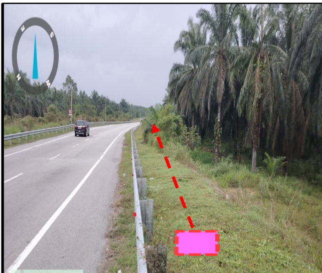
Prop New TIME MH 34 (Jln Kubu Gajah-Taiping)( 5.113198° , 100.715836° )
