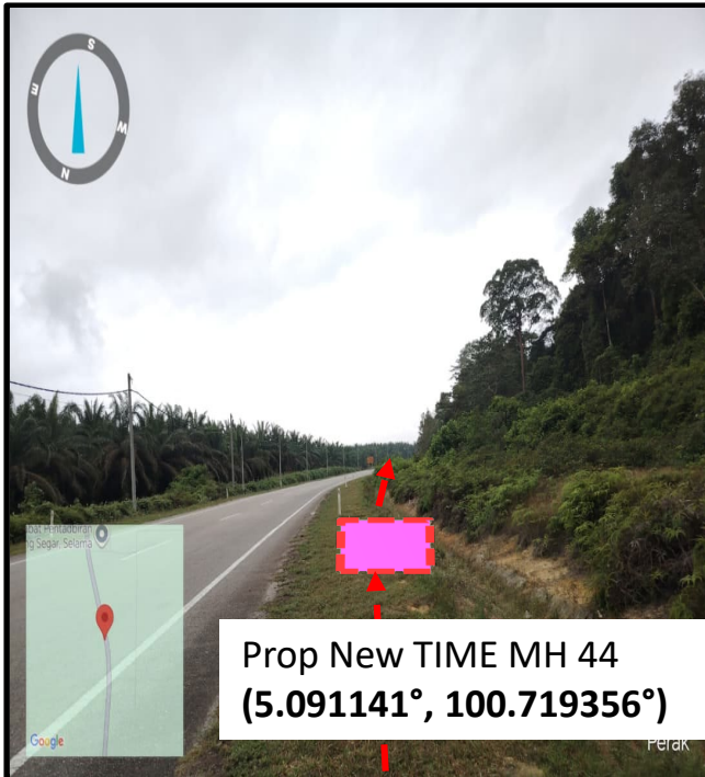
Prop New TIME MH 44 (Jln Kubu Gajah-Taiping)(5.091141°, 100.719356°)
