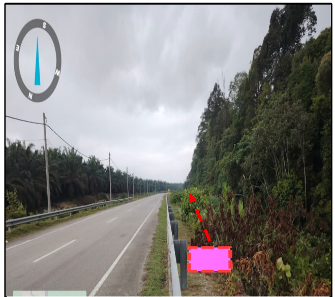
Prop New TIME MH 43 (Jln Kubu Gajah-Taiping)( 5.093391°, 100.719567° )
