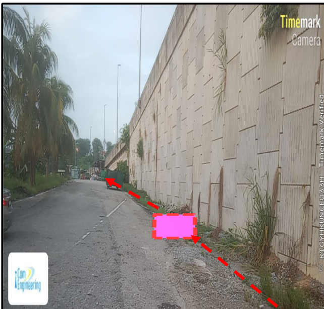
Prop New TIME MH 82 (Jln Kubu Gajah-Taiping)( 5.011412° , 100.730349° )
