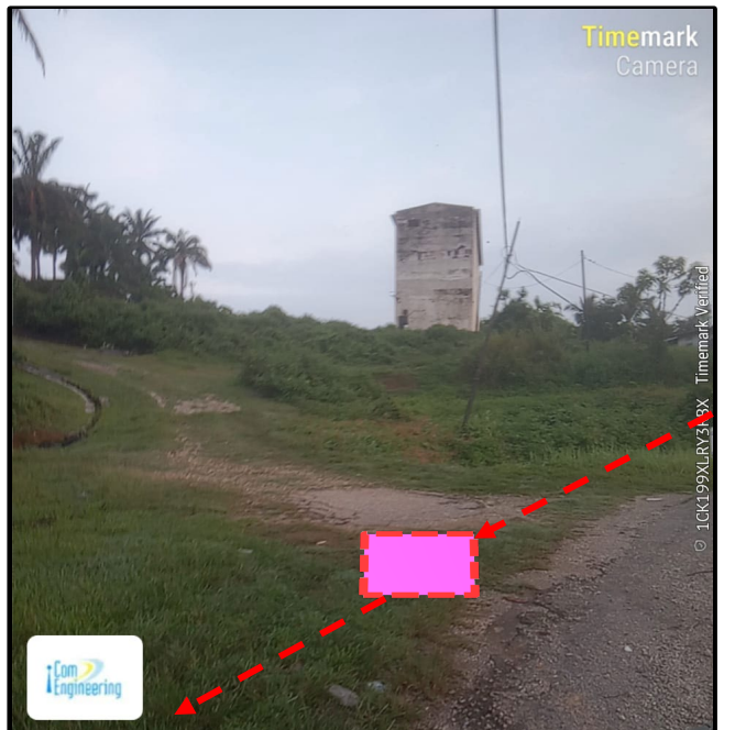
Prop New TIME MH 87 (Jln Kubu Gajah-Taiping)( 5.001457° , 100.734510° )
