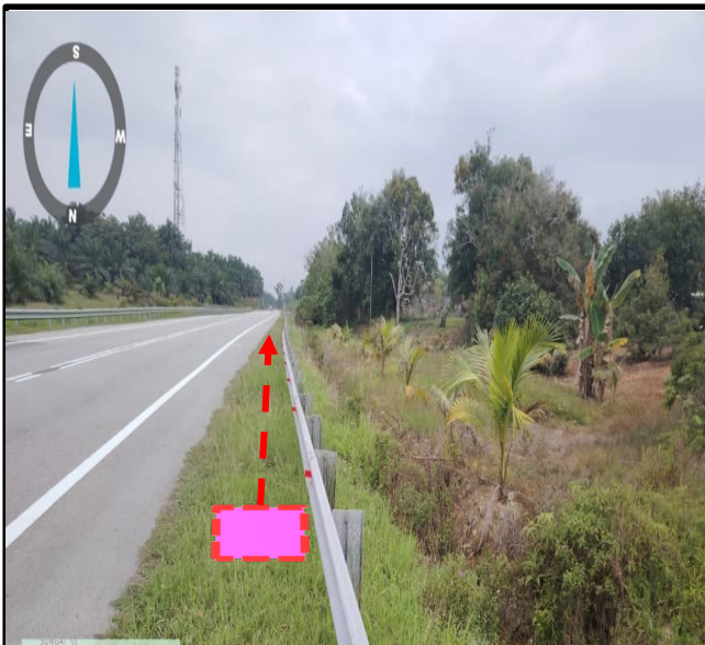
Prop New TIME MH 38 (Jln Kubu Gajah-Taiping)(5.104420°, 100.717840°)
