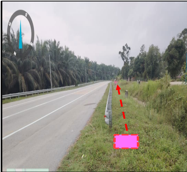
Prop New TIME MH 40 (Jln Kubu Gajah-Taiping)( 5.099941, 100.718041° )
