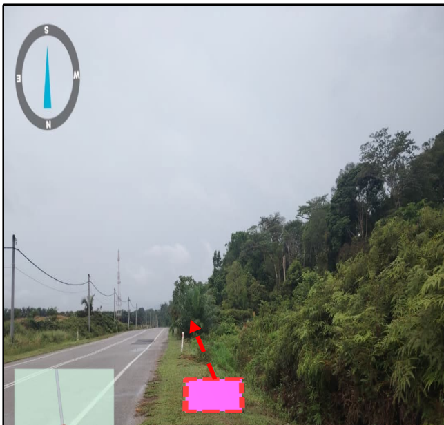
Prop New TIME MH 62 (Jln Kubu Gajah-Taiping)(5.051558°, 100.724649°)
