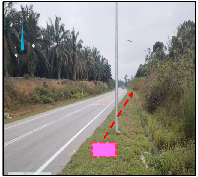
Prop New TIME MH 39 (Jln Kubu Gajah-Taiping)(5.102192°, 100.718079°)
