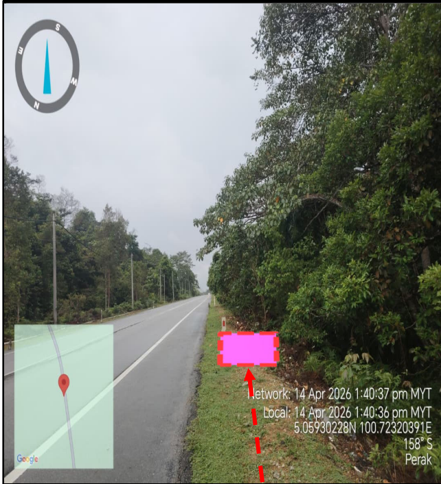
Prop New TIME MH 60 (Jln Kubu Gajah-Taiping)(5.05930228N,
