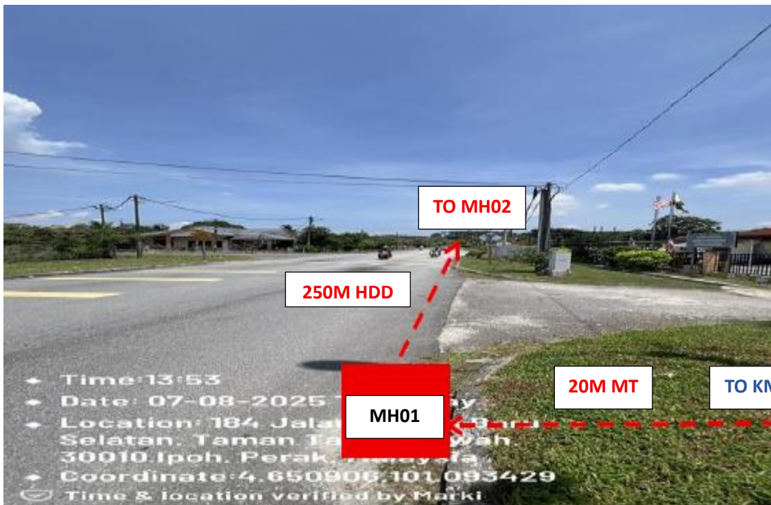
PICTURE 2 : EXISTING MH BUILDING
