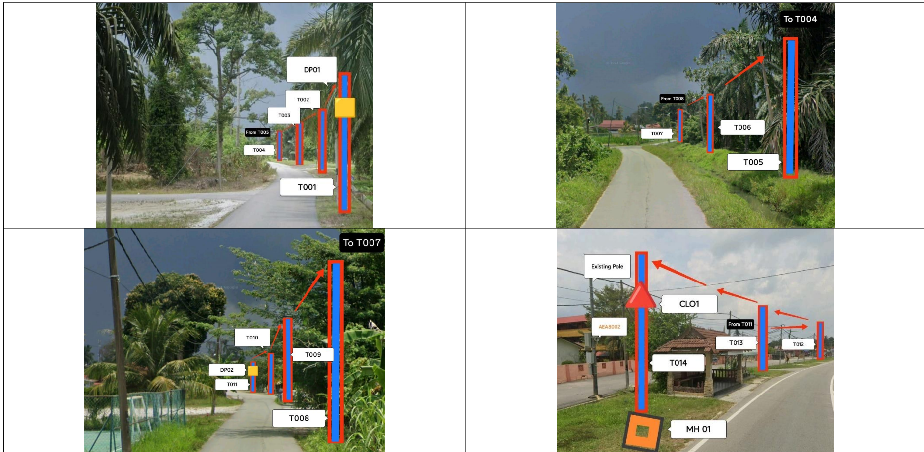
Site Photos – Proposed to install pole 7.5m
