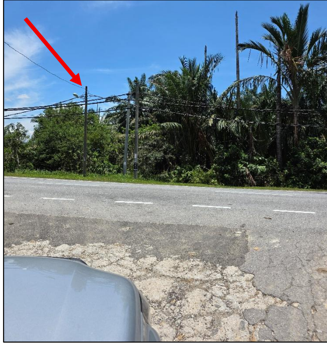
Figure 9. Propose to tap at this TNB pole (need to get permission TNB).
