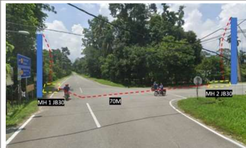
Site Photos – Proposed Manhole & HDD (Pole 7.5m for install riser)
