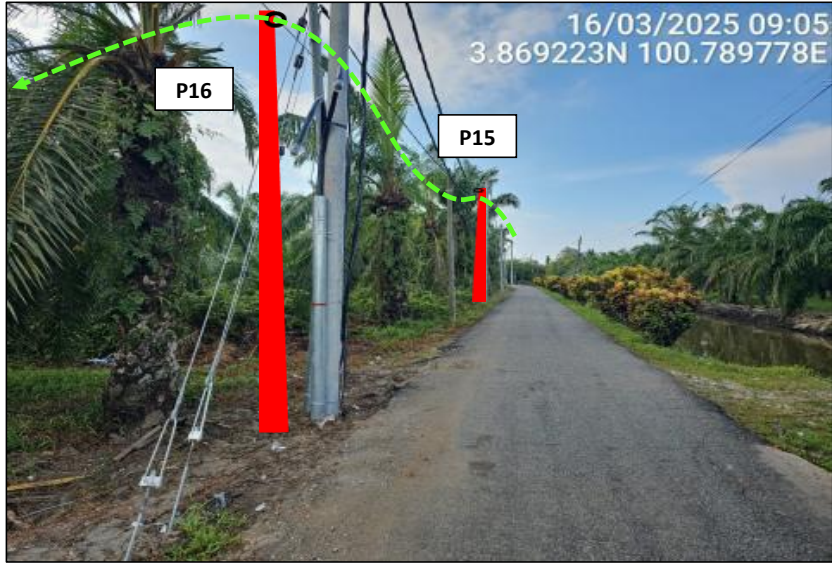
LOCATION AT UNNAMED ROAD
