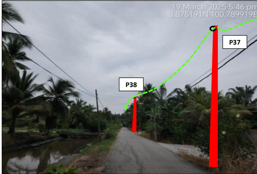
LOCATION AT UNNAMED ROAD
