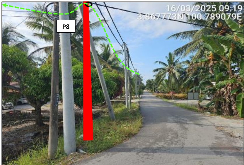
LOCATION AT UNNAMED ROAD
