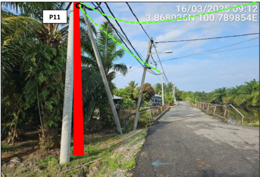
LOCATION AT UNNAMED ROAD
