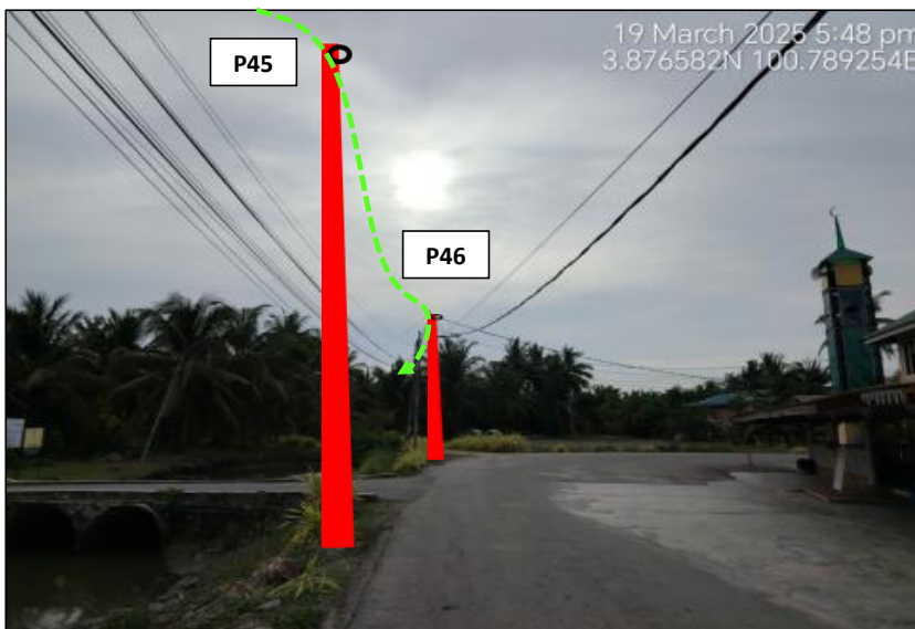
LOCATION AT UNNAMED ROAD
