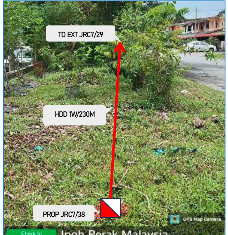
PROP JRC7/38 LOC AT JALAN DESA AMPANG 16 (ROADSIDE)
