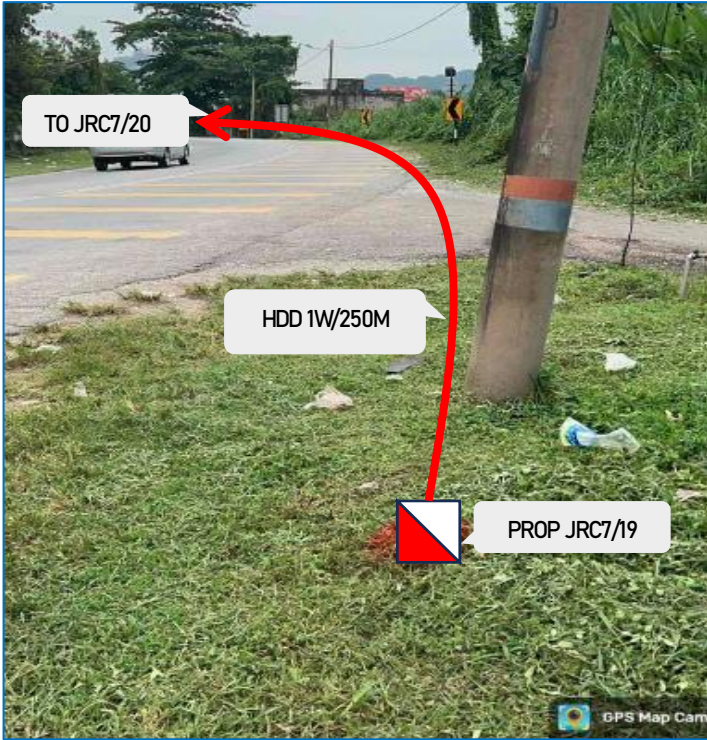
PROP JRC7/19 LOC AT JALAN AMPANG (ROADSIDE)
