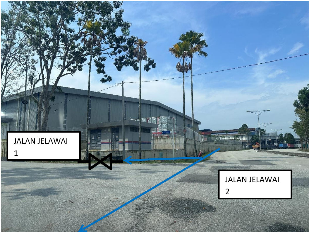
Figure 9.0 : Proposed pipeline route at Jalan Jelawai 2 and extension valve to Jalan Jelawai 1.
