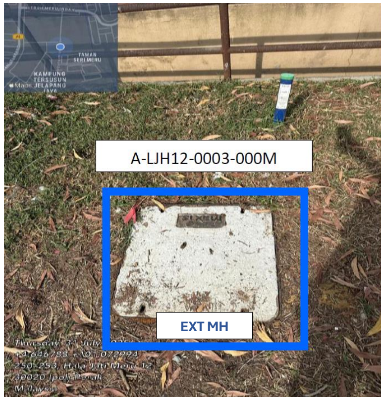
PICTURE 1 : EXISTING MAXIS MANHOLE
