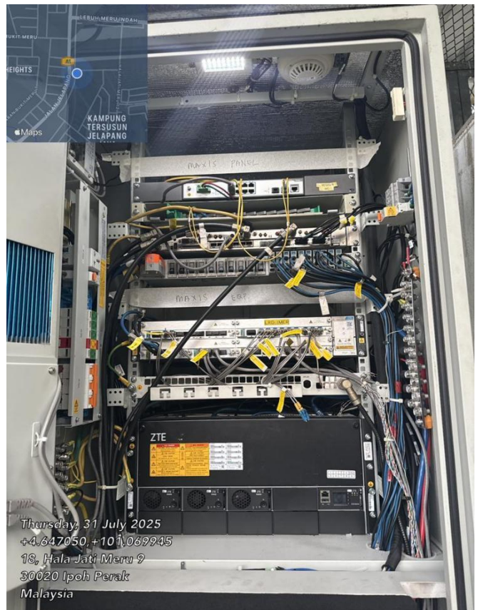
PICTURE 12 - INSIDE AREA IMER
