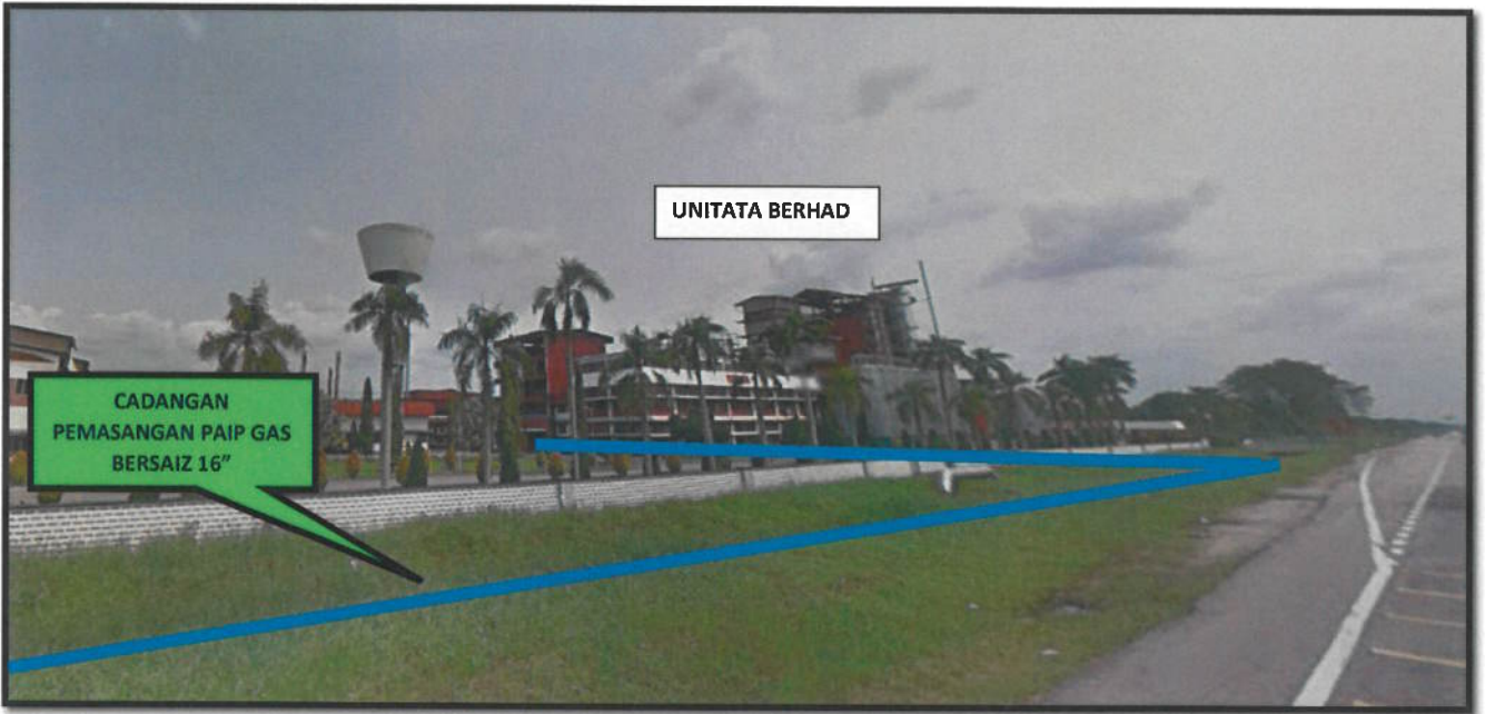
FIGURE 1.11: JALAN KLANG – TELUK INTAN (5)
