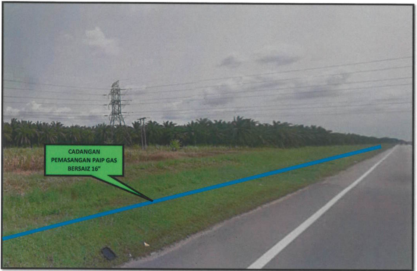
FIGURE 1.9: JALAN KLANG – TELUK INTAN (5)
