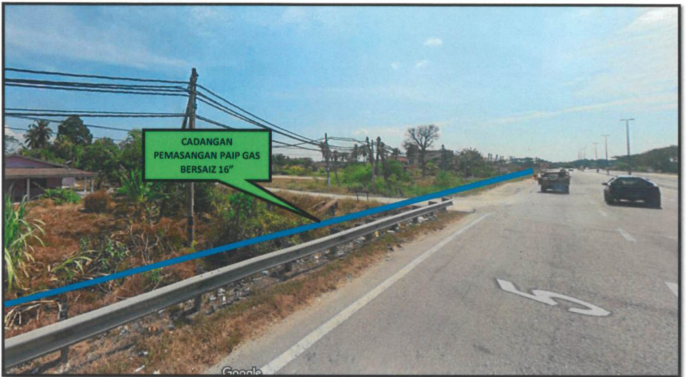
FIGURE 1.3: JALAN KLANG – TELUK INTAN (5)
