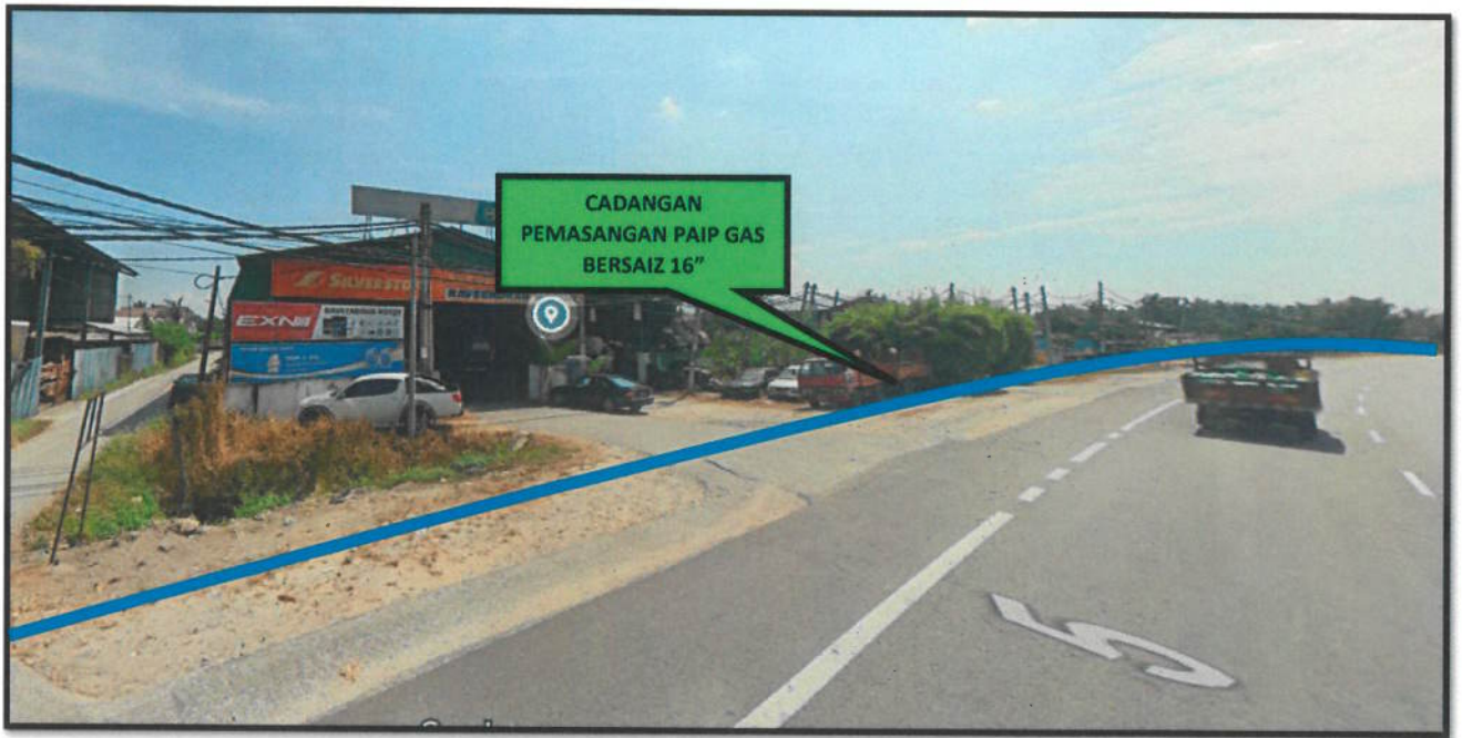
FIGURE 1.5: JALAN KLANG – TELUK INTAN (5)
