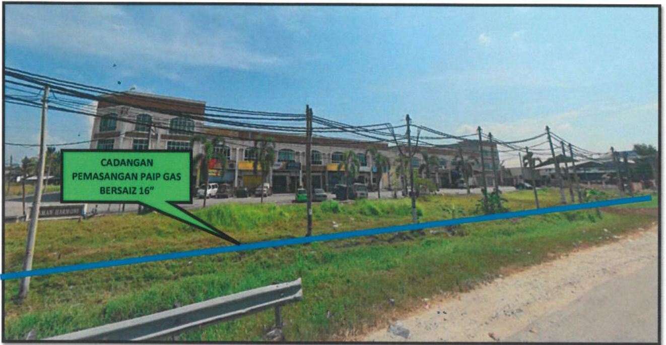
FIGURE 1.4: JALAN KLANG – TELUK INTAN (5)
