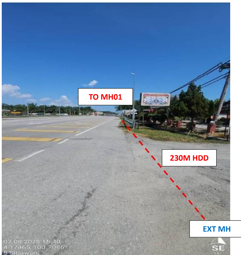
PICTURE 2 : FROM EXISTING MAXIS MANHOLE TO PROPOSE MH01
