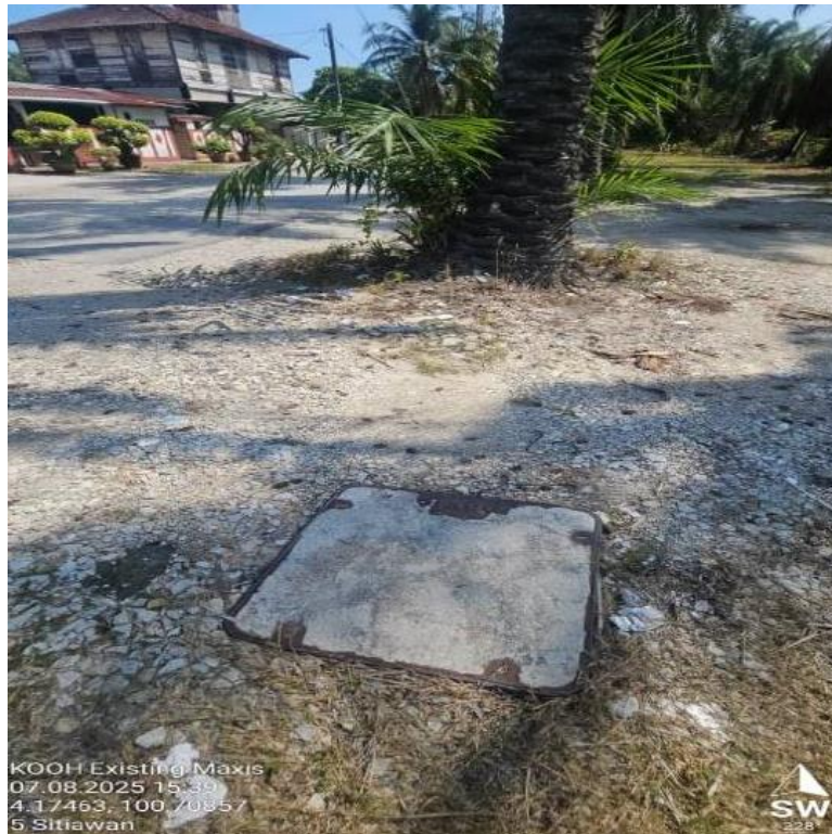
PICTURE 1 : EXISTING MAXIS MANHOLE
