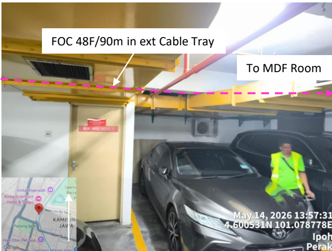
Inside Building Basement
