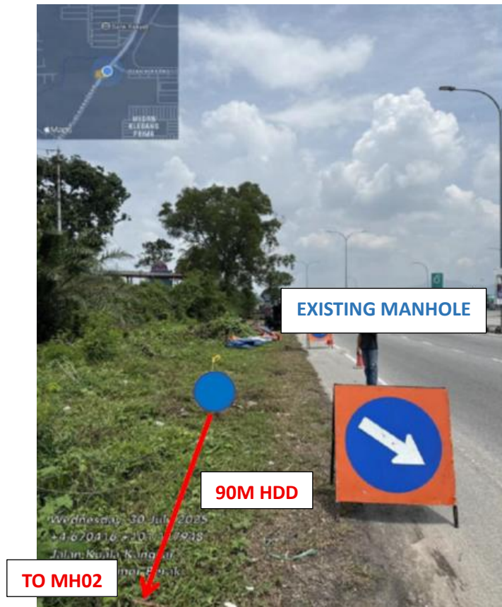
PICTURE 2 : EXISTING MANHOLE TO PROPOSE MH02
