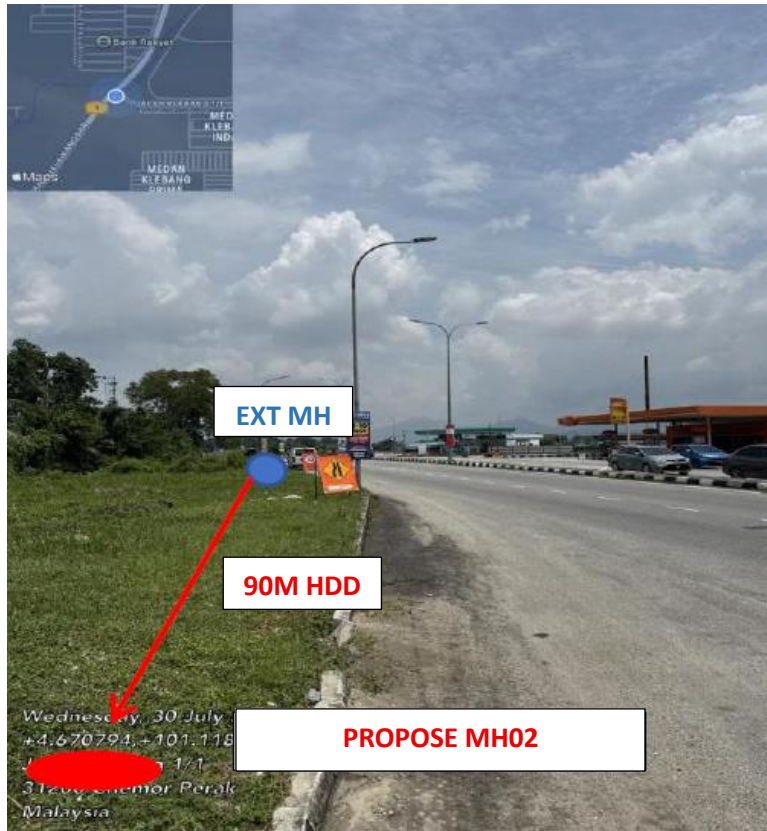
PICTURE 3 : EXISTING MANHOLE TO PROPOSE MH02
