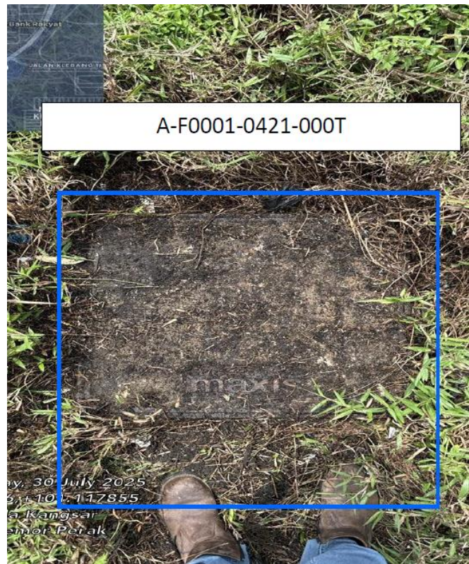
PICTURE 1 : EXISTING MAXIS MANHOLE
