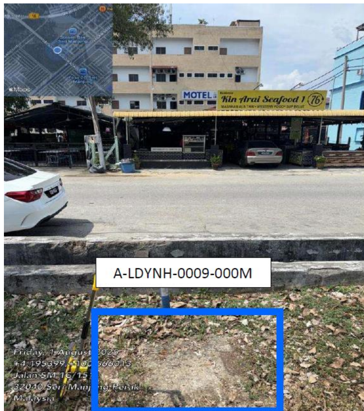
PICTURE 1 : EXISTING MAXIS MANHOLE
