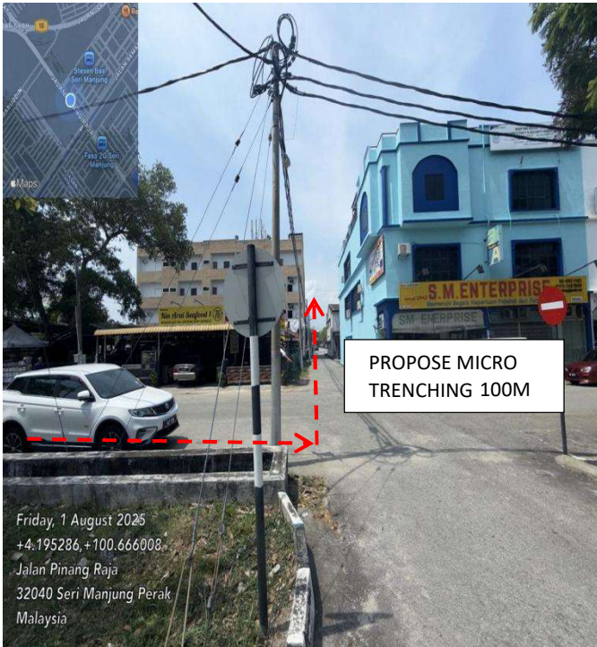
Picture 3 - JALAN SM 1C/15
