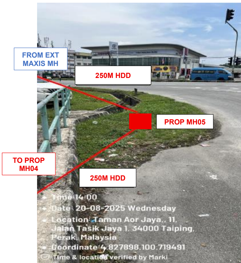
PICTURE 2 : HDD 250M TO PROP MH05
