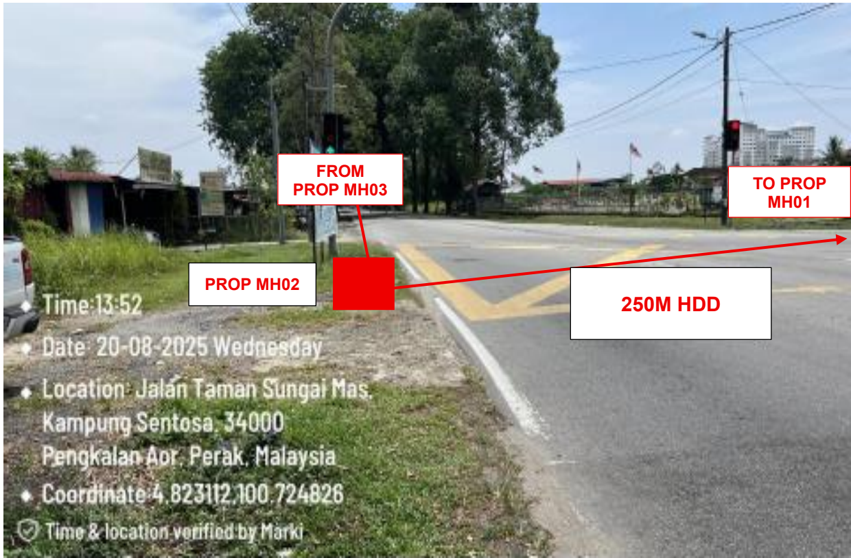
PICTURE 5 : HDD 250M TO PROP MH02
