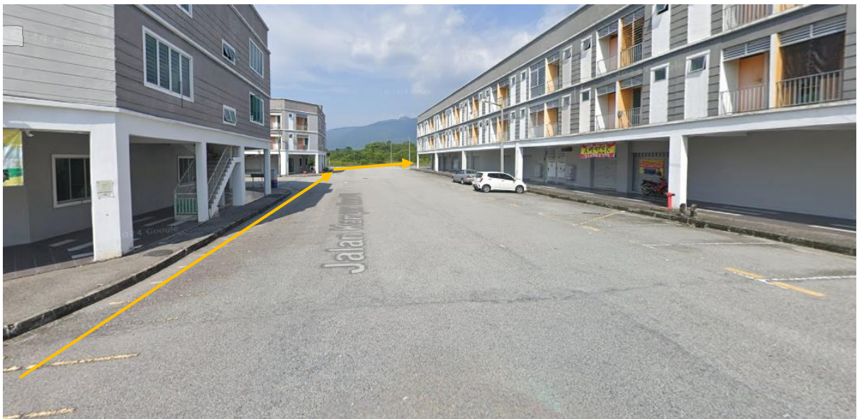
KERJA – KERJA OPEN CUT JALAN BERTURAP (98M) JALAN KAMPAR BARAT 10 (4.322002, 101.129705, 4.322587, 101.130616)
