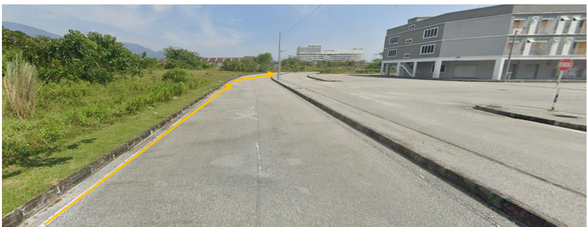
KERJA – KERJA OPEN CUT JALAN BERTURAP (61M) JALAN KAMPAR BARAT (4.322587, 101.130616, 4.321905, 101.130823)
