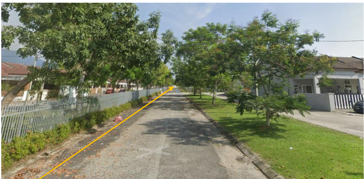
KERJA – KERJA OPEN CUT JALAN BERTURAP (364M) JALAN PUTRA BERLIAN 9 (4.321394, 101.131271, 4.31876, 101.133335)
