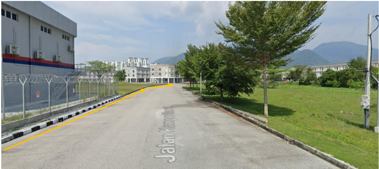
KERJA – KERJA OPEN CUT JALAN BERTURAP (303M) JALAN KAMPAR BARAT 9 (4.321902, 101.127538, 4.322002, 101.129705)
