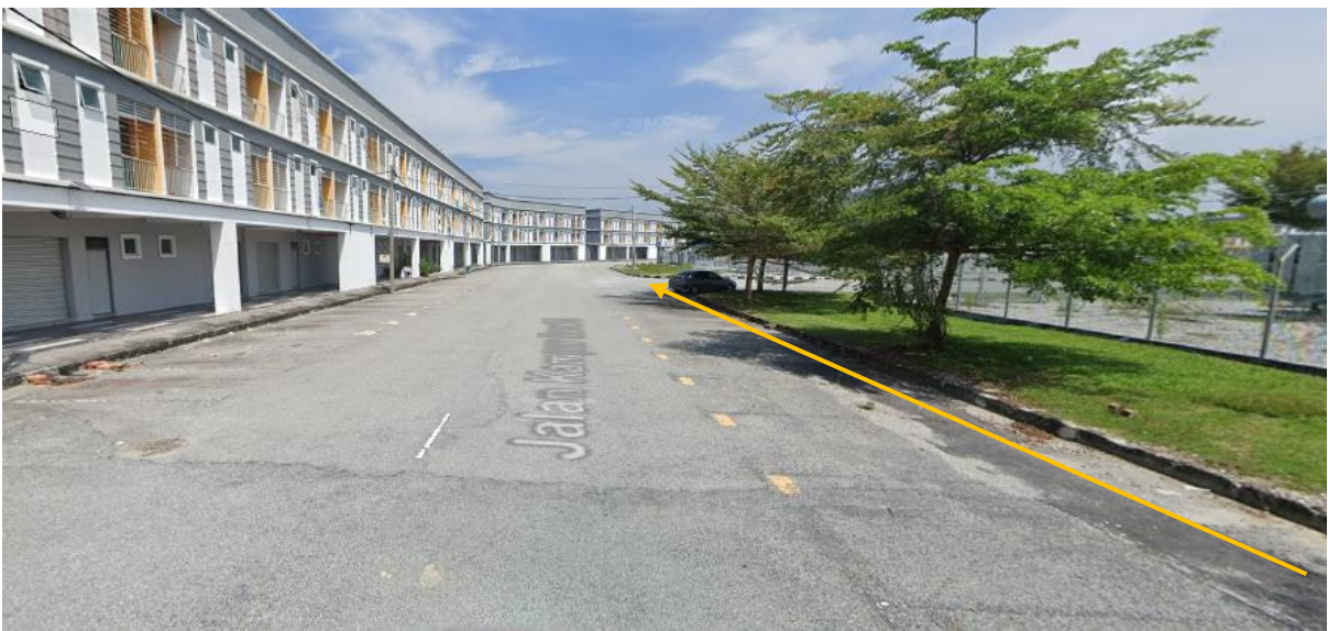
KERJA – KERJA OPEN CUT JALAN BERTURAP (40M) JALAN KAMPAR BARAT 9 (4.321693, 101.127672, 4.321902, 101.127538)
