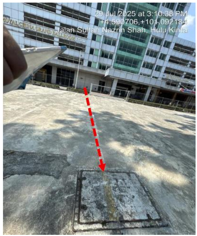
PICTURE 2 : EXISTING MH BUILDING
