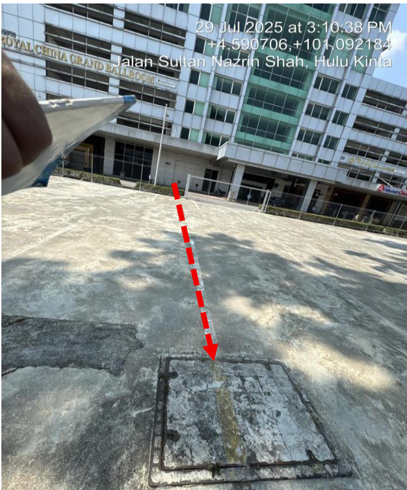
Picture 3 – EXISTING MH BUILDING
