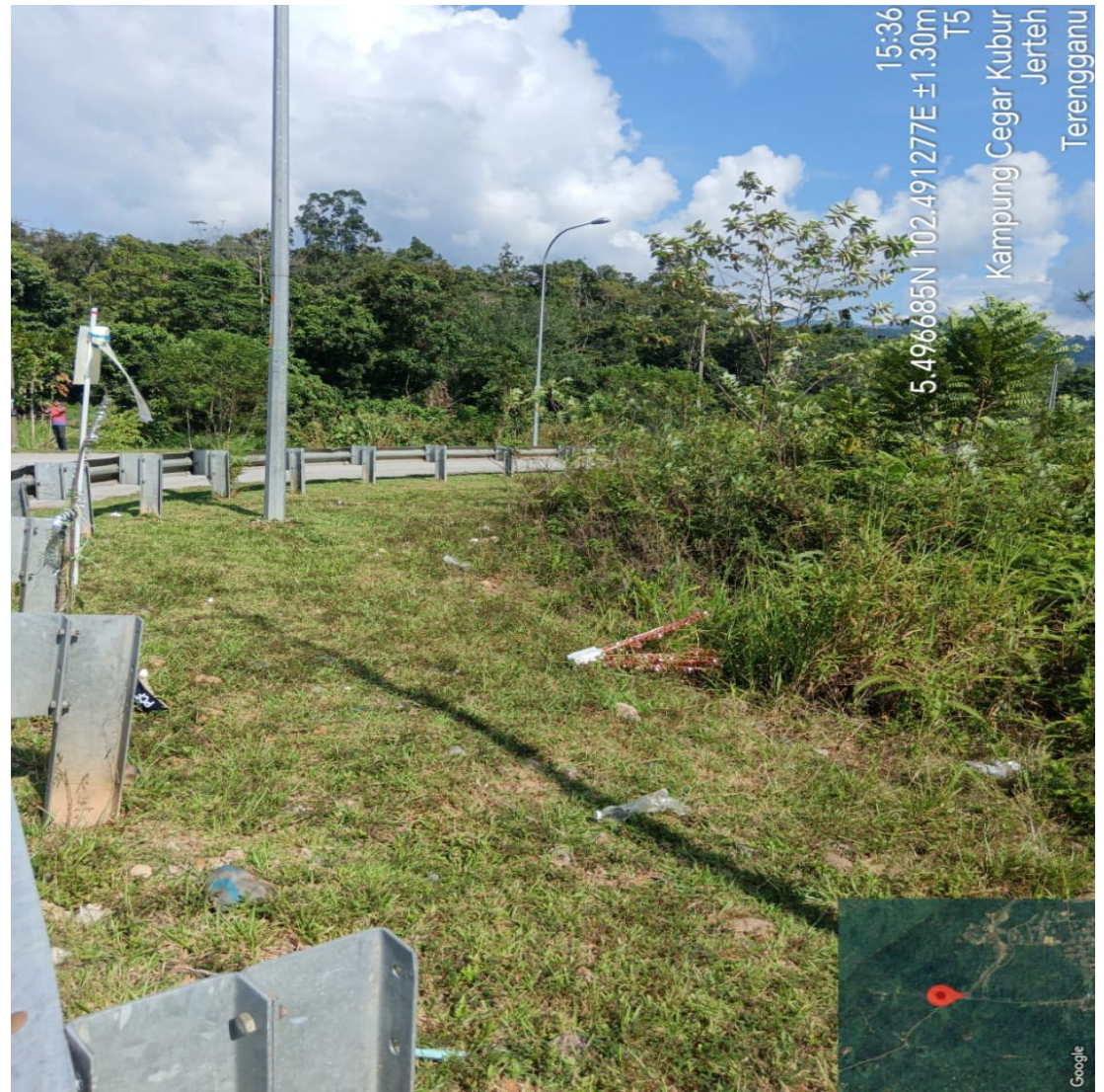
END POINT NEW JRC7 MANHOLE
