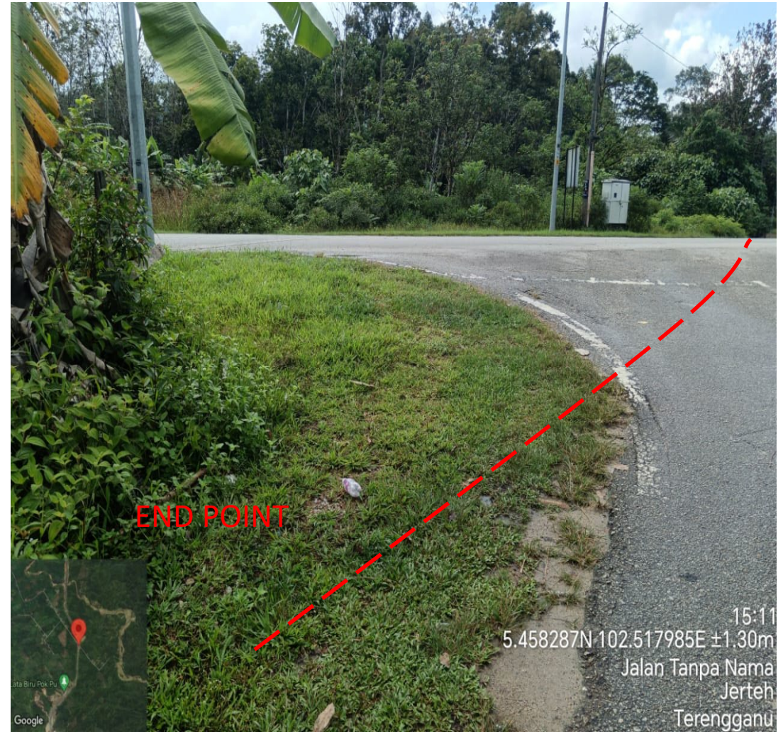
END POINT NEW JRC7 MANHOLE
