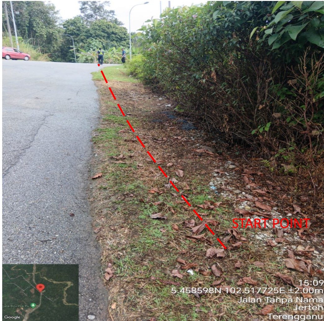
START POINT NEW JRC7 MANHOLE
